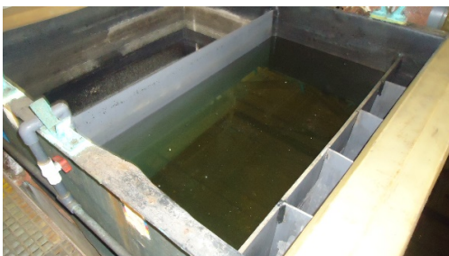
Photo #13 – Out of service zinc plating solutions stored in the large barrel line tanks.
