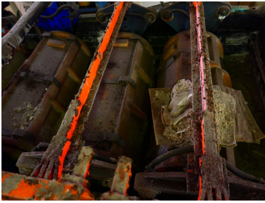
Photo #7 – Rusted out of service zinc plating large barrel line equipment.
