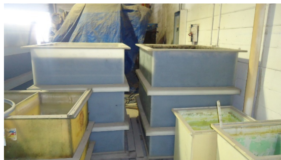
Photo #25 – Hazardous plating waste containers staged for wastewater treatment system.
