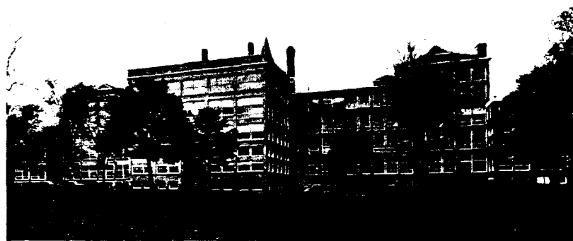
General view of the large Niagara Falls plant of National Biscuit Company. White lead proves highly economical for such industrial paint maintenance
