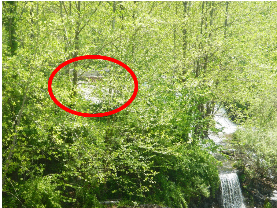
Figure 2. Same view as Figure 1 but zoomed in. Facility structures visible behind trees (red circle).
