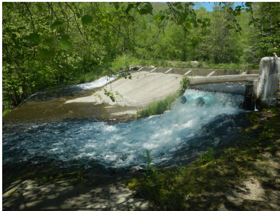
Figure 3. Facility water intake structure. Overflow seen is source of new discharge. This water has no contact with any trout ponds.
