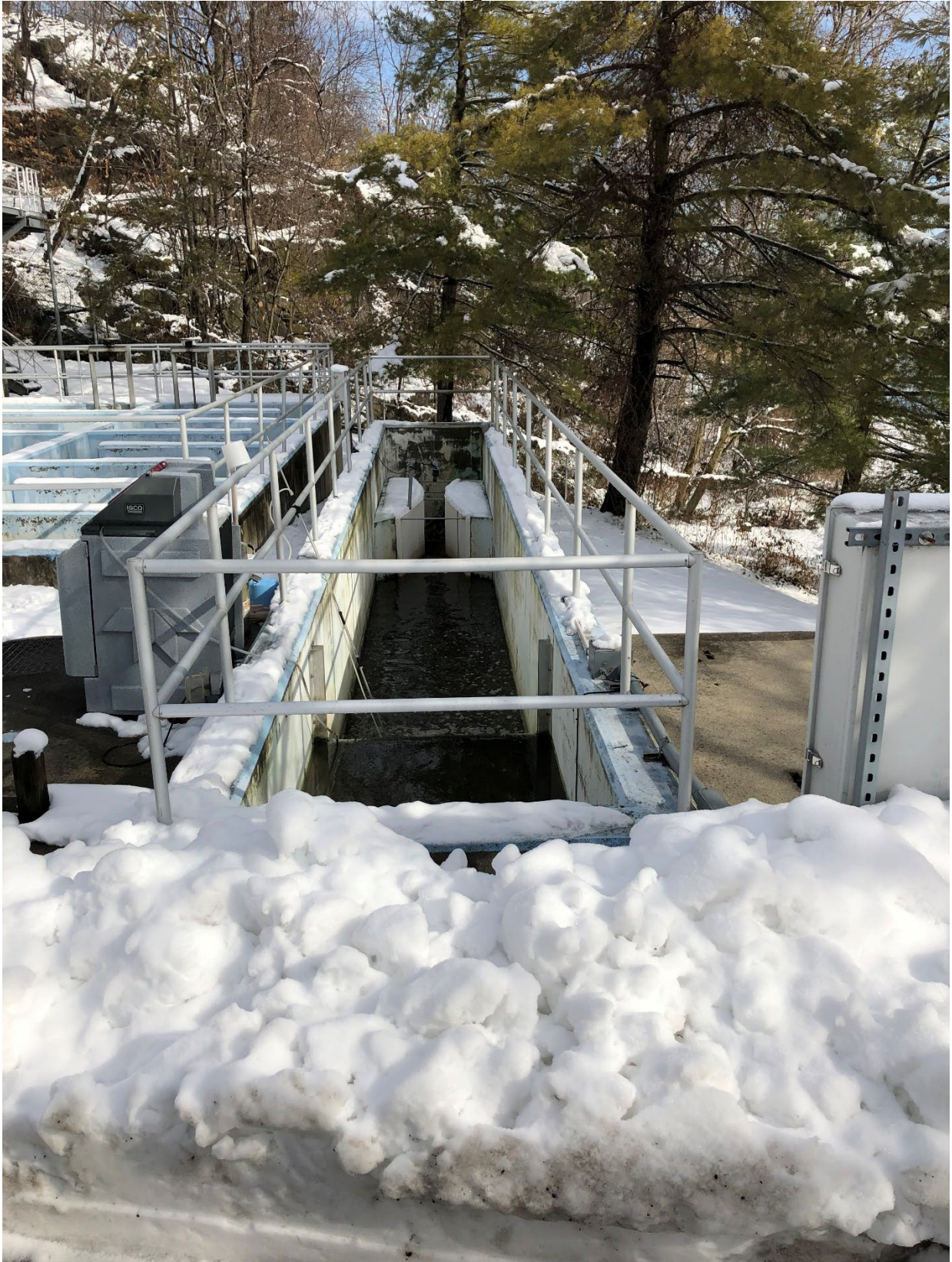
Photo #2: Another view of the effluent sampling location.
