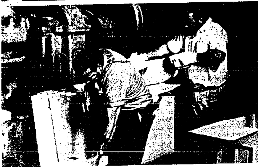
Two asbestos workers cutting block. Relatively little dust is dispersed into the air . . .
