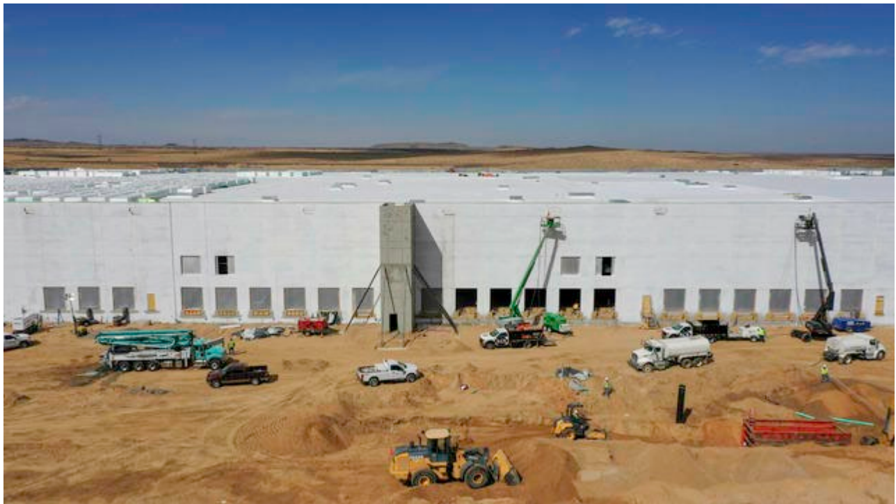
The Amazon fulfillment center under construction in Los Lunas from Roberto E. Rosales/Journal, February 23, 2022.
