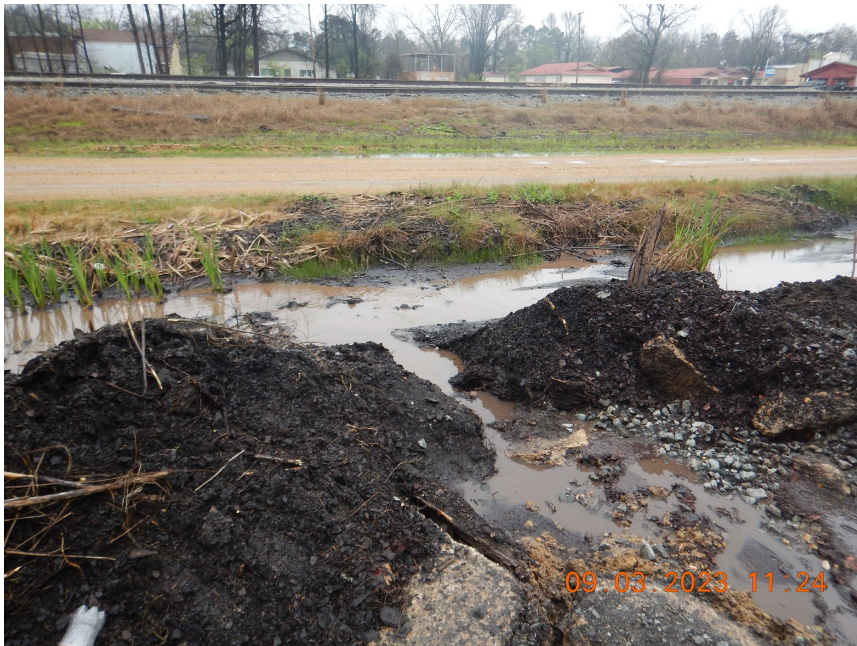
Photograph within the Bearden facility upgradient of the railway access and roadway. Note: the debris and the run-off into an open earthen lined conduit. (DSCN2484) Photographed by C. Sherwood
