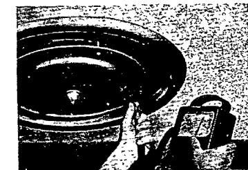
BALANCING —Single air stream allows direct velocity reading of volume immediately.
