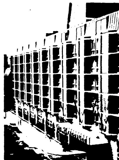
The Gloucester Hotel, West London, where lead adhesively bonded to hardboard is used for roof fascia and to cover a rooftop mechanical penthouse.
