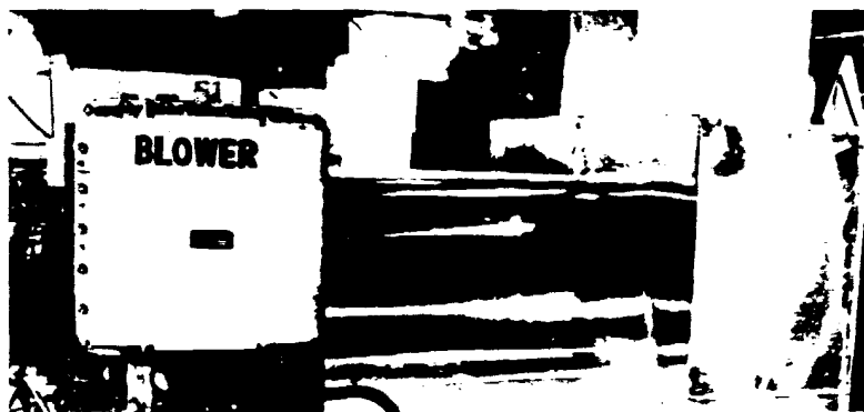
Sheet lead, glass fiber and aluminum reduced sound levels near this blower by more than eight decibels.
