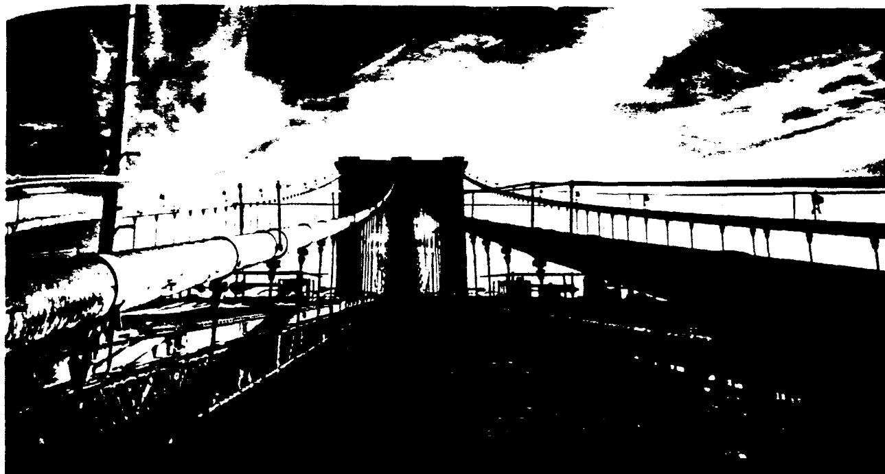
Dramatic view of upper level of bridge before painting.
