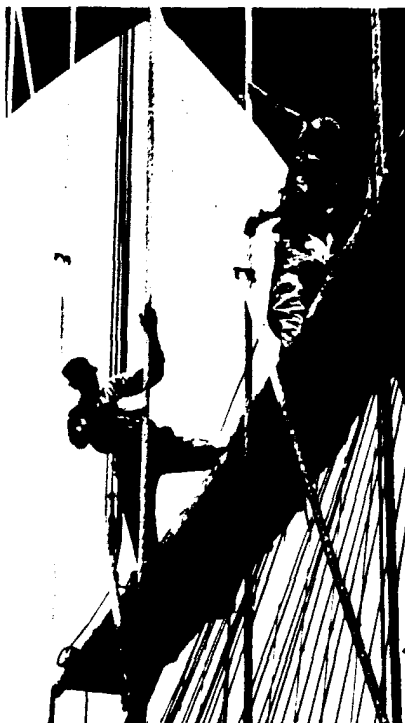
Vertical cabling of Brooklyn Bridge was painted silver.
