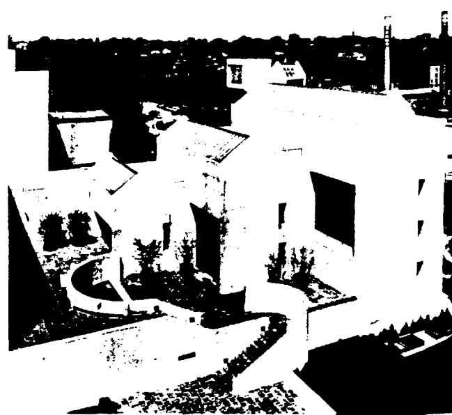
The use of TCS provided one of the architectural highlights for the three-tier roof of a group of buildings designed for the New York Bar Association Center, Albany, N.Y.
