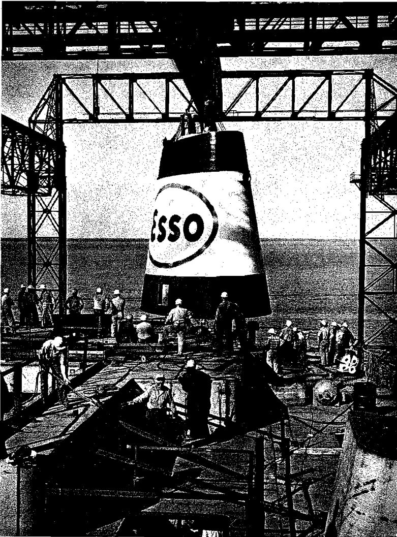
One of the last items to be installed on the ESSO BOSTON was her teardrop-shaped stack. It is 29 feet in height and 27'6" in length. The distance from the keel to the top of the stack is equal to the height of an eleven-story building.
