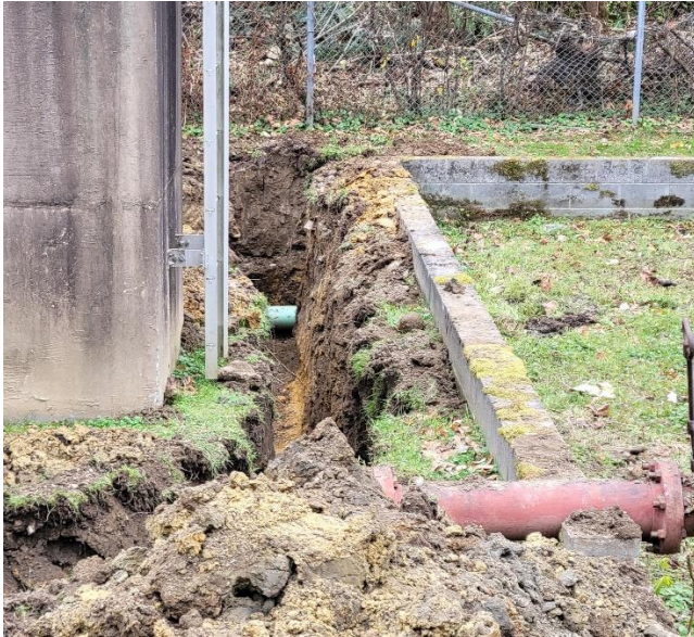
Photo 7. Trench used to replace WAS line.
