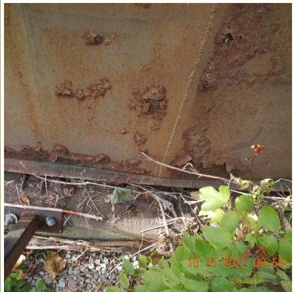
Photos 9 and 10. Exterior side wall of the package plant. Presence of corrosion.
