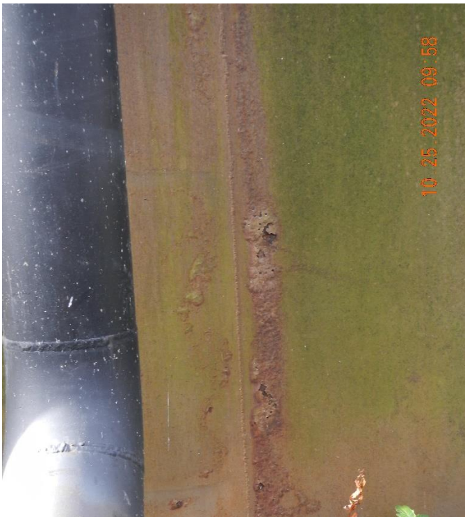
Photos 9 and 10. Exterior side wall of the package plant. Presence of corrosion.
