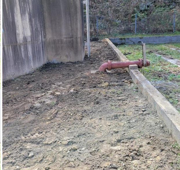
Photo 8. After WAS line replacement.
