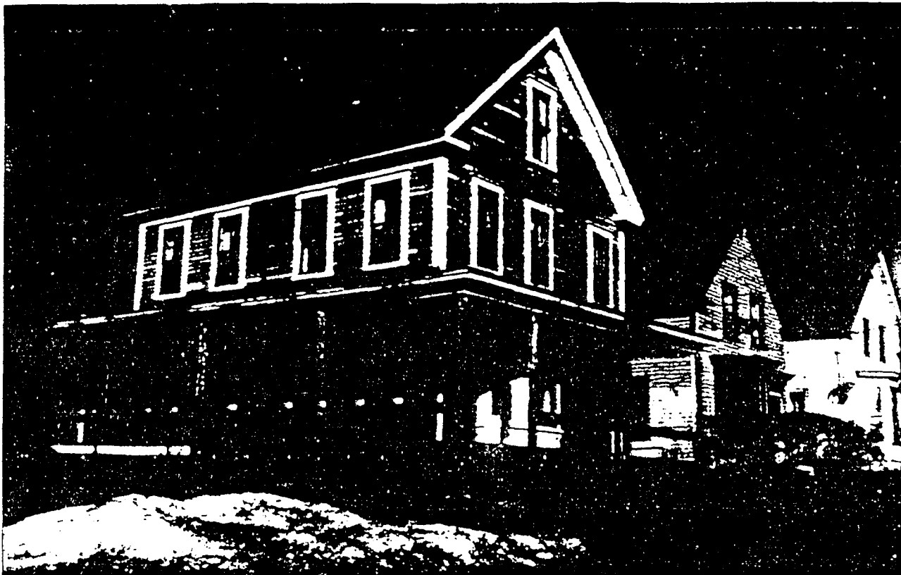
When Sandra and Lee Roseberry bought this Farmington, New Hampshire house in 1983, they did not know that the paint on the exterior walls contained 51 percent lead.
