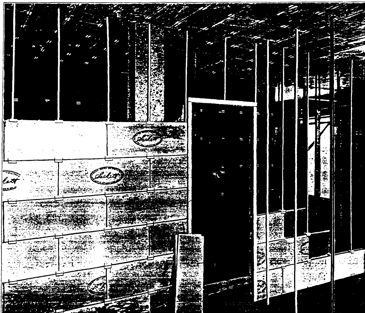
Jester-Sackett Hollow Partition under construction. Minimum thickness (plastered) 2\frac{3}{4} ". Partition can also be constructed in 3", 3\frac{1}{2} ", 4", 5" or 6". Use \frac{3}{8} " Sackett Plaster Board 18"x 32". Note also Jester-Sackett Suspended Ceilings.
