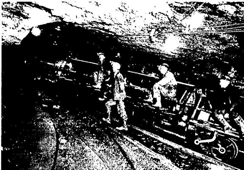
A safety man-trip on a 20-degree haulage slope. Haulage is still a serious source of accidents in coal mines.
