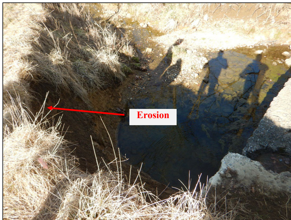
Photograph 4. Site for Potential Floodplain Restoration BMP: (DSCN2829) Additional view of observed streambank erosion.
