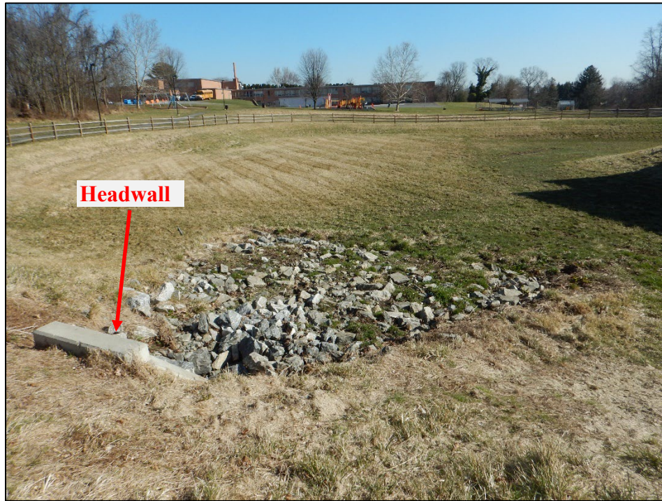
Photograph 7. Kensington Club Basin Rehabilitation Project: (DSCN2836) View, facing northeast, of the detention basin. Note the inflow headwall in the left side of the photo.
