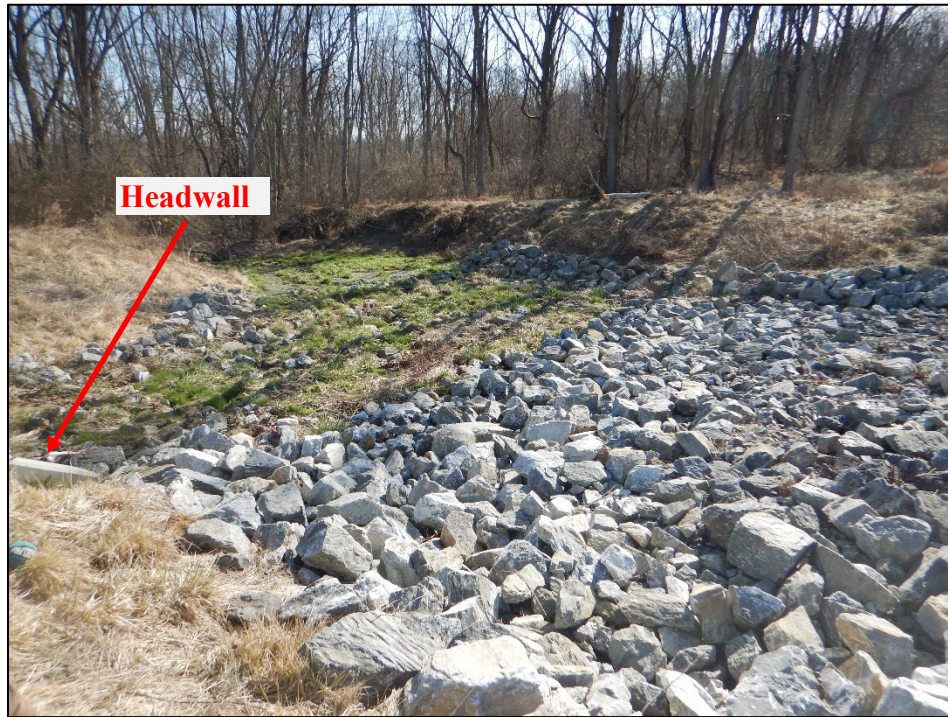
Photograph 13. Kensington Club Basin Rehabilitation Project: (DSCN2844) View, facing east, of the armored emergency spillway, basin outflow headwall, and drainage area towards an unnamed tributary to the Conestoga River.
