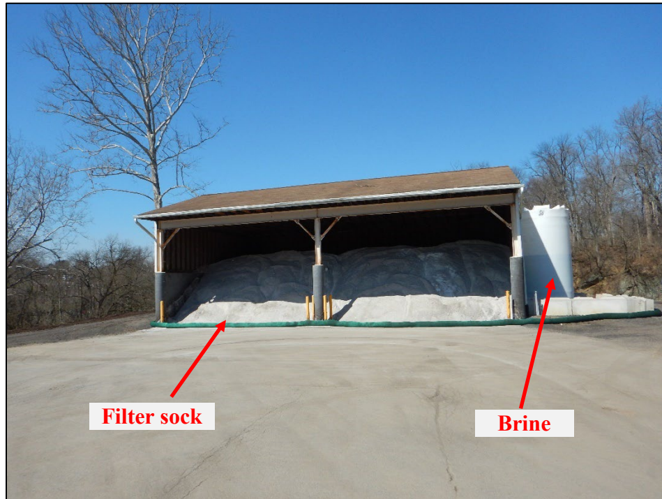
Photograph 31. Township Public Works Campus: (DSCN 2910) View, facing north, of the Campus's salt storage building, attached to the upper garage. The building was enclosed on three sides and had a filter sock placed along the open side. There was no observed salt migration from the building from the building. Note the Campus' brine storage on the right side.
