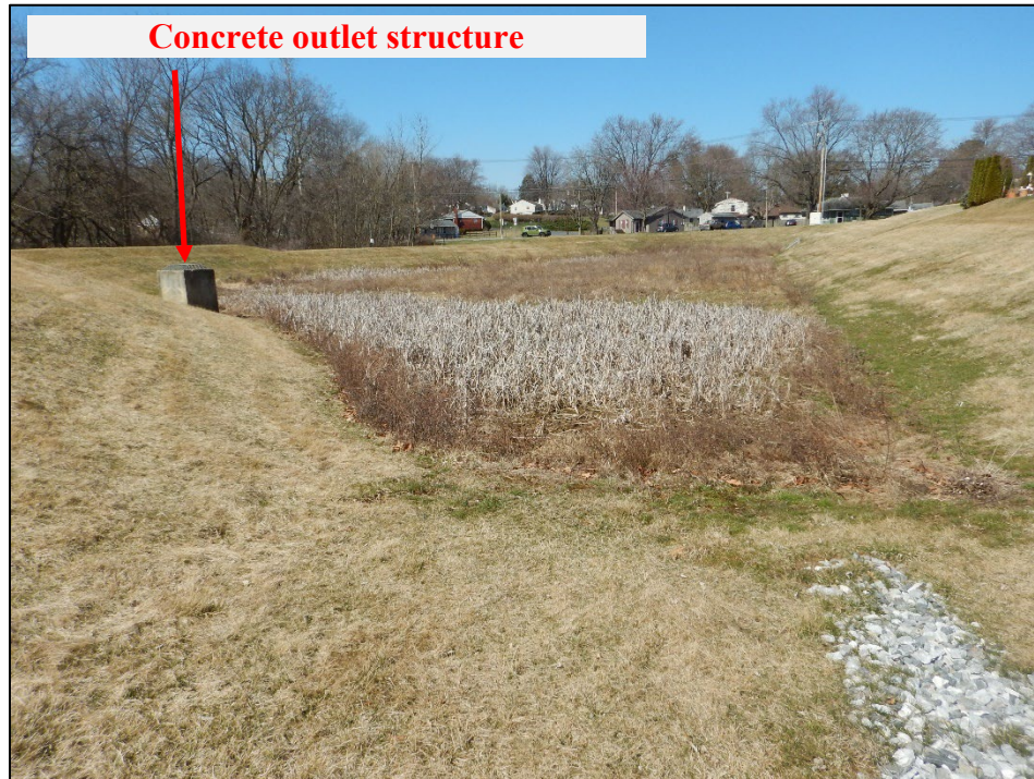
Photograph 25. Southern Village Detention Basin: (DSCN2885) View, facing northwest, of the detention basin and concrete outlet structure. The basin appeared to be well maintained.
