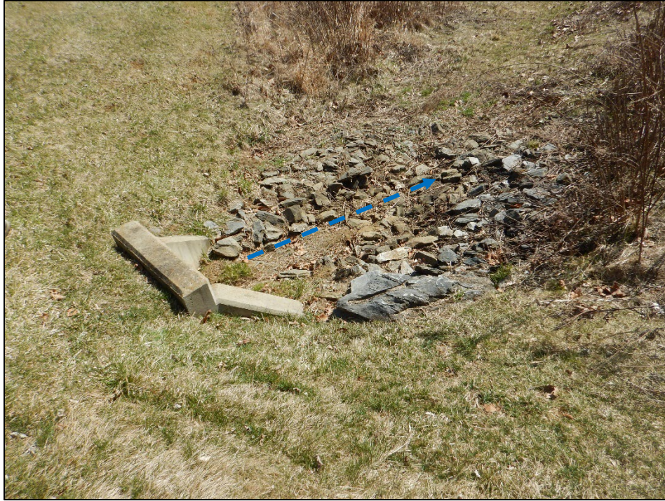
Photograph 27. Southern Village Detention Basin: (DSCN2890) View of the basin’s outflow headwall and drainage area that conveys stormwater to an unnamed tributary of the Conestoga River. Note the blue arrow indicating the direction of flow.
