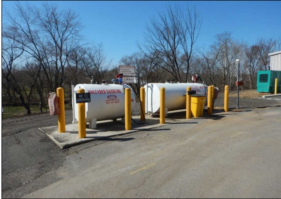
Photograph 33. Township Public Works Campus: (DSCN2909) View, facing northwest, of the two aboveground fuel tanks (one 1,000-gallon diesel, one regular 500-gallon unleaded gasoline). The EPA Inspection Team observed spill kits in the adjacent building.
