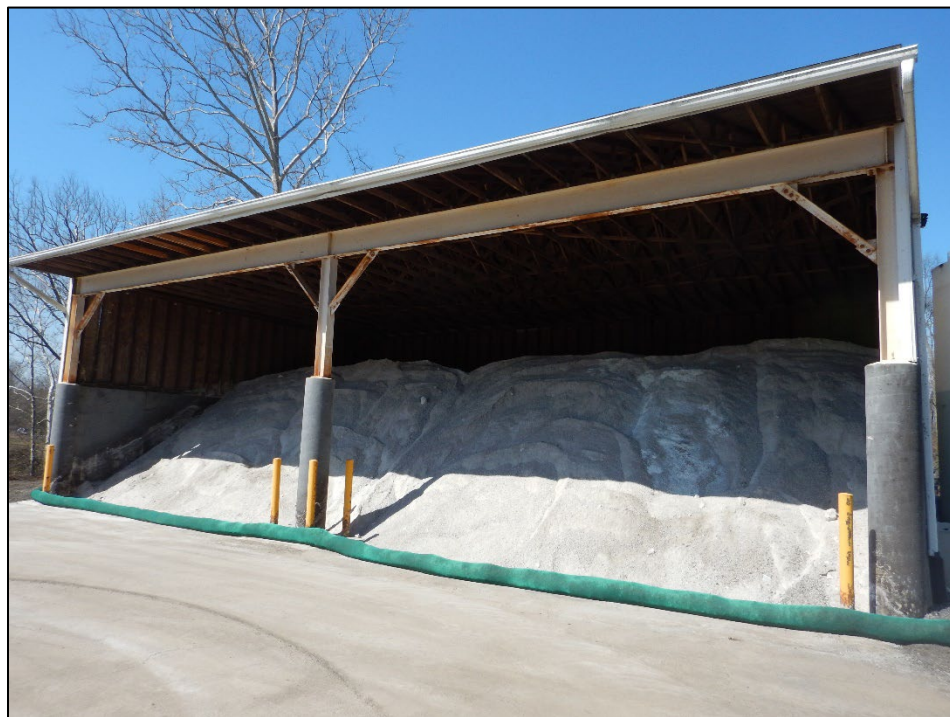
Photograph 32. Township Public Works Campus: (DSCN 2911) Closer view of the salt storage building and filter sock, as shown in Photograph 31.
