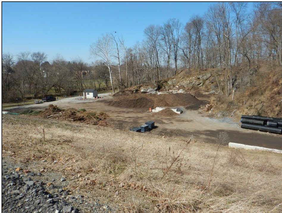
Photograph 34. Township Public Works Campus: (DSCN2914) View, facing northwest, of the Township's wood waste recycling center that also serves as material and aggregate storage.
