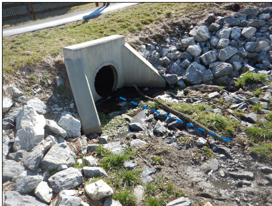
Photograph 8. Kensington Club Basin Rehabilitation Project: (DSCN2838) Closer view of the inflow headwall and pipe, as shown in Photograph 7. Note the blue arrow indicating the direction of flow.
