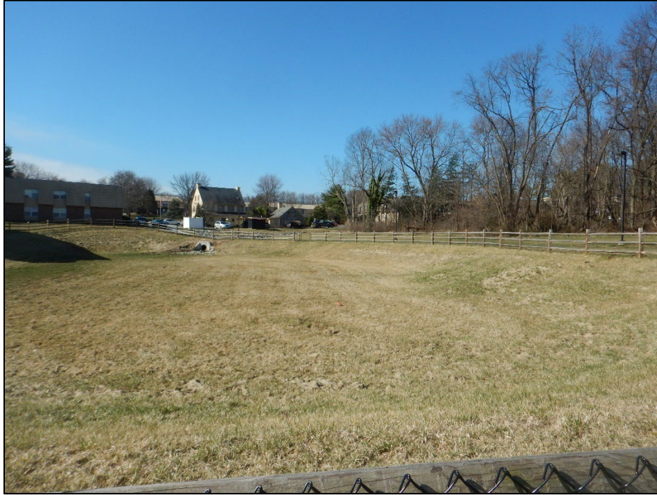
Photograph 9. Kensington Club Basin Rehabilitation Project: (DSCN2840) Additional view, facing west, of the basin that was observed to be mowed and largely trash free at the time of the inspection.
