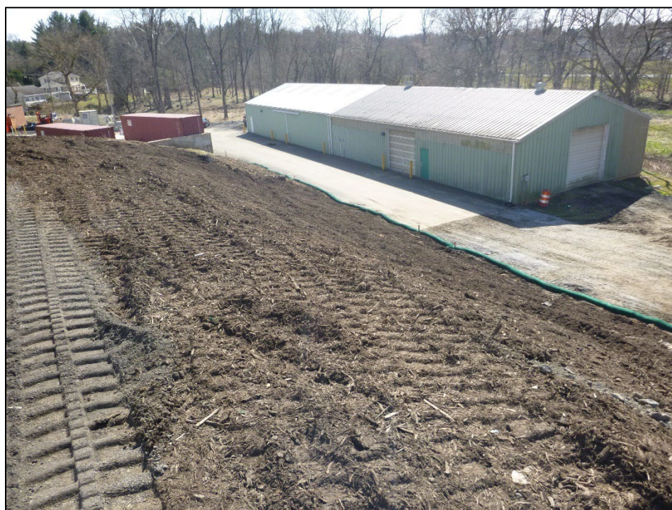
Photograph 40. Township Public Works Campus: (P1060610) View, facing west, of the lower garages at the Campus primarily used for vehicle and materials storage.
