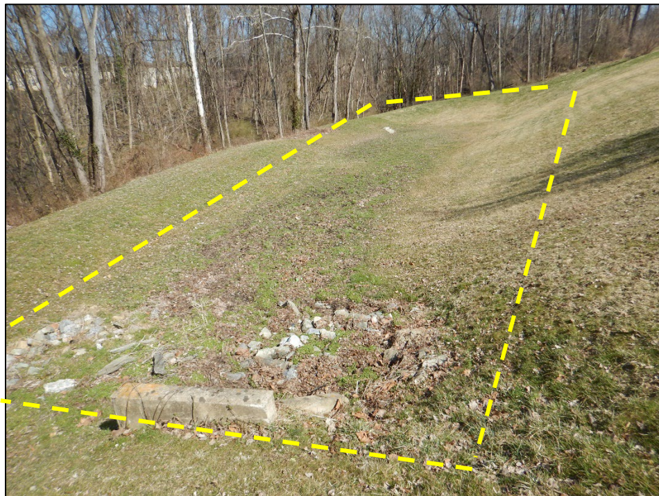
Photograph 18. Chadwick Circle Detention Basin: (DSCN2864) View, facing northeast, of the basin. The basin was mowed and largely free of trash and debris. Note the yellow dotted lines indicating the approximate boundary of the basin.
