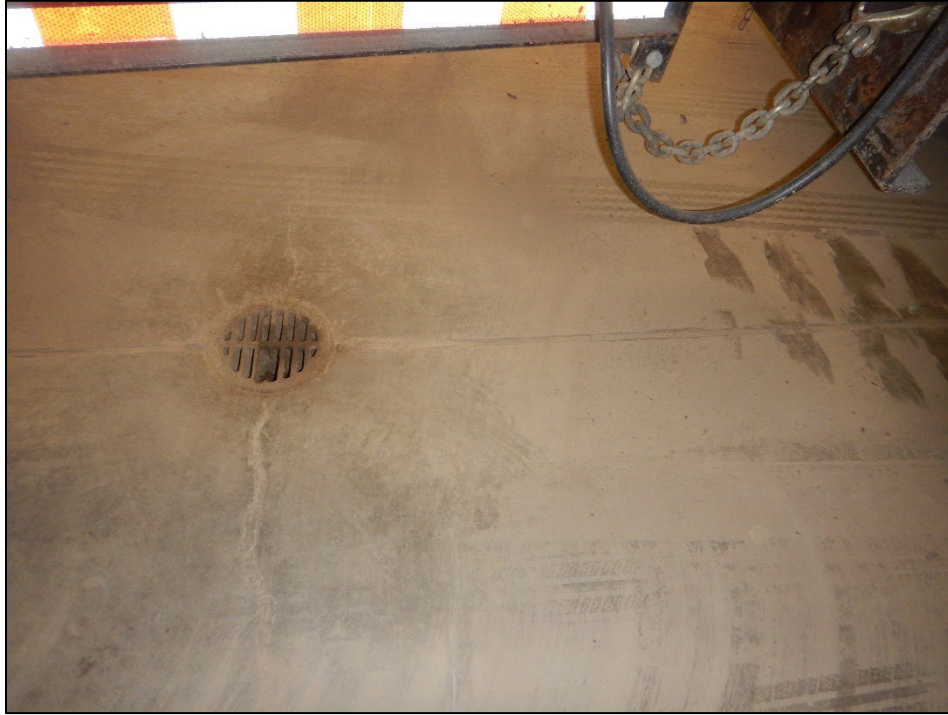
Photograph 41. Township Public Works Campus: (DSCN2934) View of one of the two (2) floor drains located in the lower garage. At the time of the inspection, Township representatives were unsure as to what these drains were connected to.
