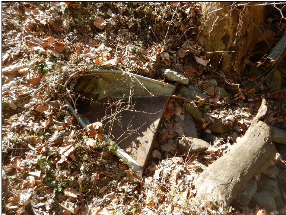
Photograph 20. Chadwick Circle Detention Basin: (DSCN2873) View of the basin's outlet pipe that conveys stormwater to a vegetated ravine that flows into the Gable Park Basin.
