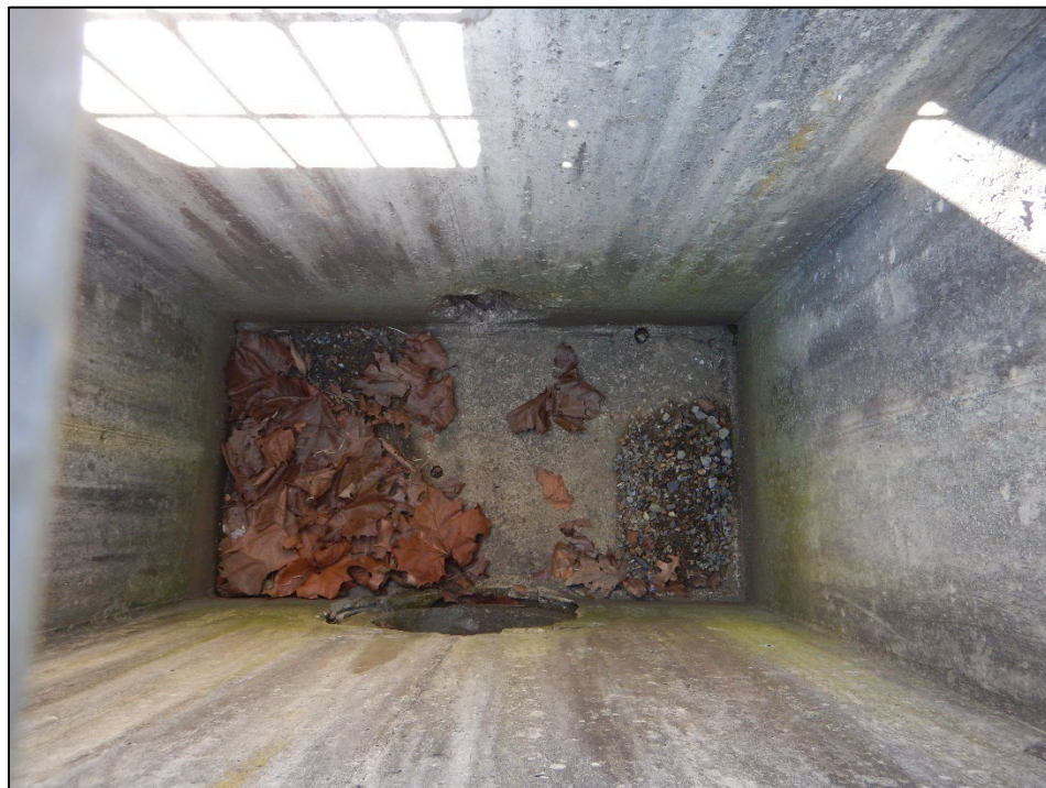
Photograph 26. Southern Village Detention Basin: (DSCN2888) View inside the basin's outlet structure, as shown in Photograph 25. There was no observed trash or flow at the time of the inspection.
