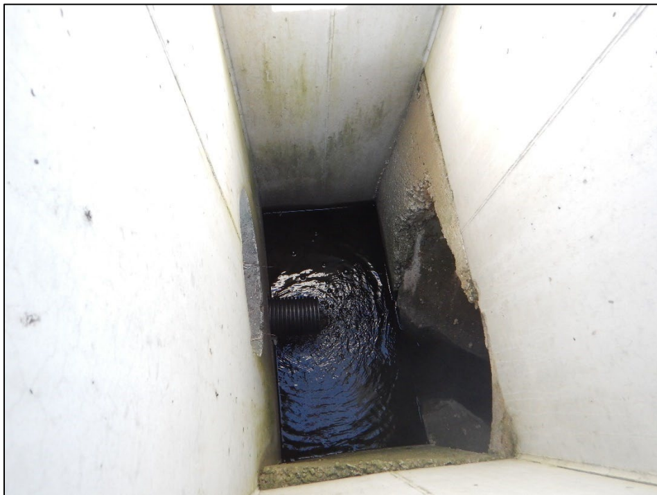
Photograph 12. Kensington Club Basin Rehabilitation Project: (DSCN2849) View inside the basin's concrete outlet structure as shown in Photographs 10 and 11. There was no observed trash inside the outlet structure, and the Township representative stated there were groundwater sources contributing to the observed flow.
