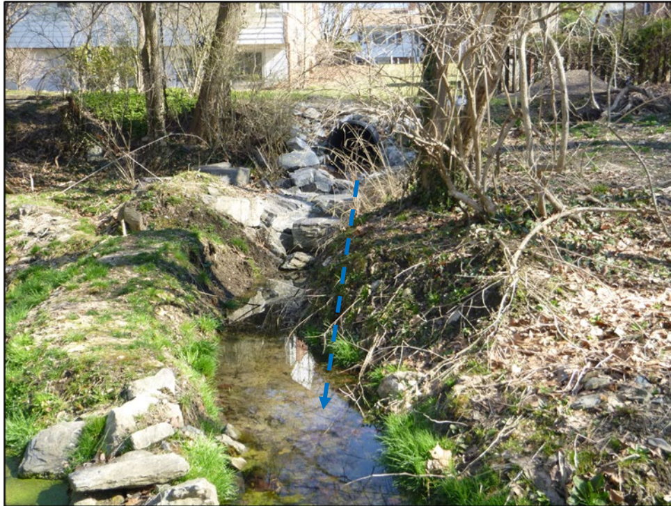
Photograph 15. Springhouse Road Swale: (P1060574) Closer view of the swale's inflow pipe and main channel, as shown in Photograph 14. Note the blue arrow indicating the direction of flow.
