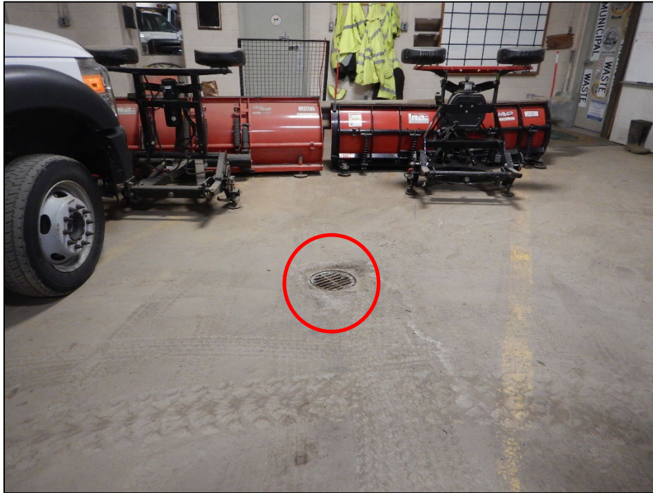
Photograph 37. Township Public Works Campus: (DSCN2921) View, inside the upper garage, of a floor drain connected to an underground OWS which then conveys to the City of Lancaster’s sanitary sewer.
