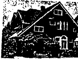
AFTER: Styling this home with SWP Modern Brown was truly successful and now it will not show the effects of weathering.
