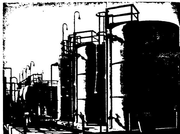
Above, some of the tanks that will be used for the storage of caustic, hydropolymer, and sulphuric acid
