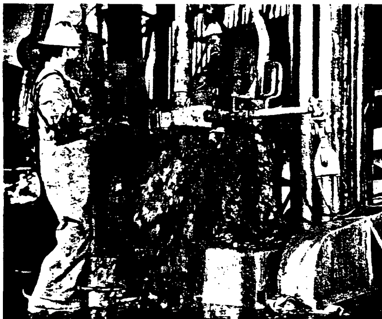
Sulphur and oil are found in the same type of salt dome deposit. Core samples obtained by this sulphur drilling team will help engineers to determine the extent and quality of the brimstone formation
