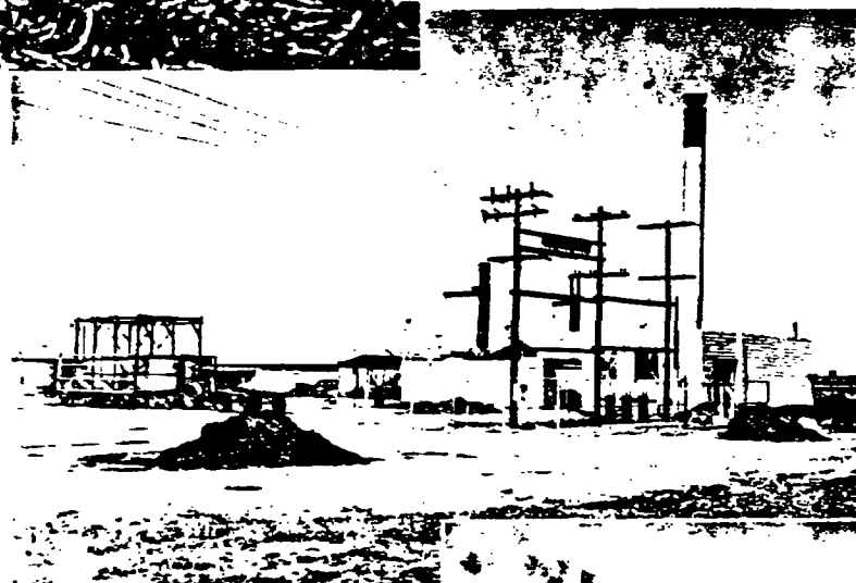
Three common sights in the Indiana mint country: Above, harvested much like hay, the mint is cut and afterwards is loaded by machine... Right, one of the many stills whose black-topped smokestacks tower above the low-lying mucklands. ... Right, below, arrived at a still, the mint is compressed into vats where the oil is steamed out of the leaves
