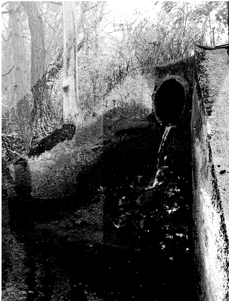
Hawley: Outfall located on the northeast end of Hawley Avenue near Ezra Street. Sample point is indicated by a red "x".
