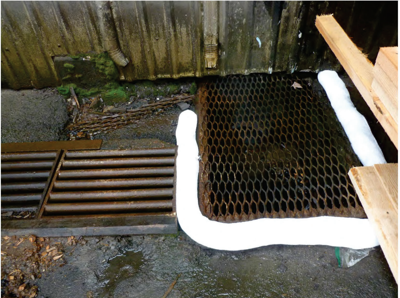
Photo 5 / P1000820 – Catch Basin, with filter sock
