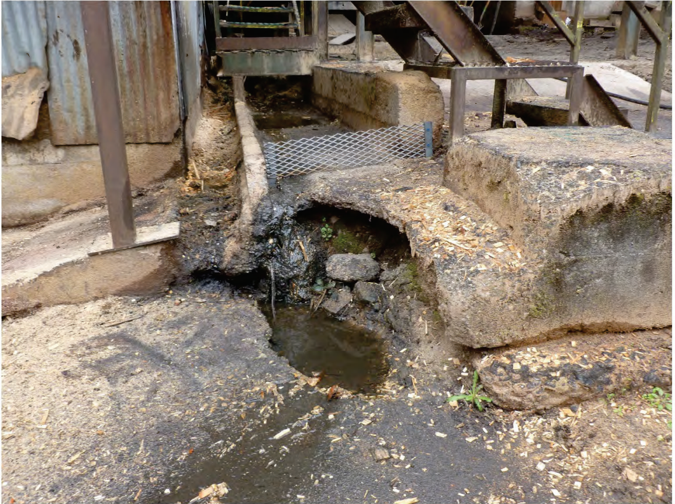
Photo 13 / P1000828 – Outflow from Roof
