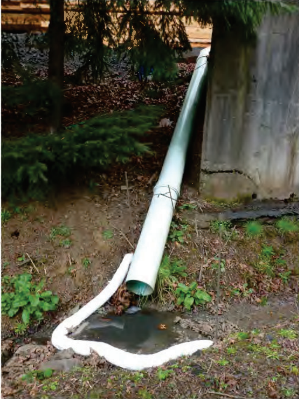
Photo 10 / P1000825 – Drain, east side
