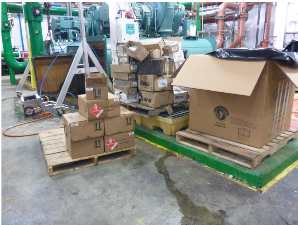
Photo 22: Area within Main CAA where wastes are consolidated according to color-coding system. The cubic yard box and some smaller containers are open. None of the containers are labeled as hazardous waste, marked with an accumulation start date, or identified with an indication of the hazards of their contents.
