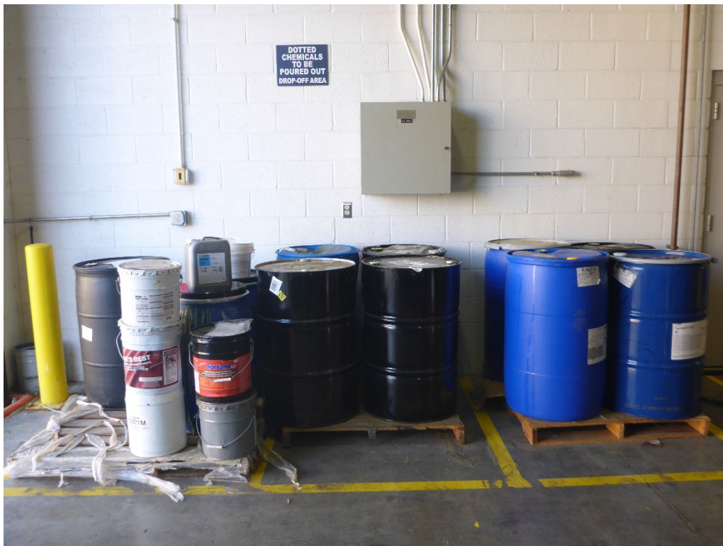
Photo 24: Row of containers along the wall just to the left when entering the Main CAA. None of the containers were labeled as hazardous waste, and many were not marked with an accumulation start date or identified with an indication of the hazards of their contents.
