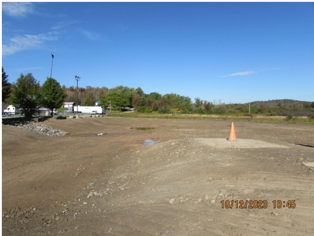
IMG 1625: View facing north showing R-2. The cone sits atop the holding tank that takes flow from inside the building and is set to remain in place.
