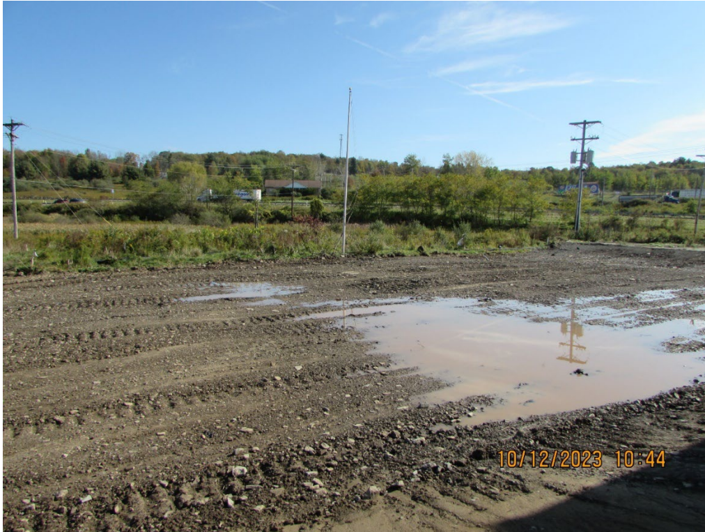
IMG_1622: View facing slightly southeast, up-gradient of R-1. At the time of the inspection, sections of R-1 were holding water and was observed to be draining east towards the Unnamed Tributary.
