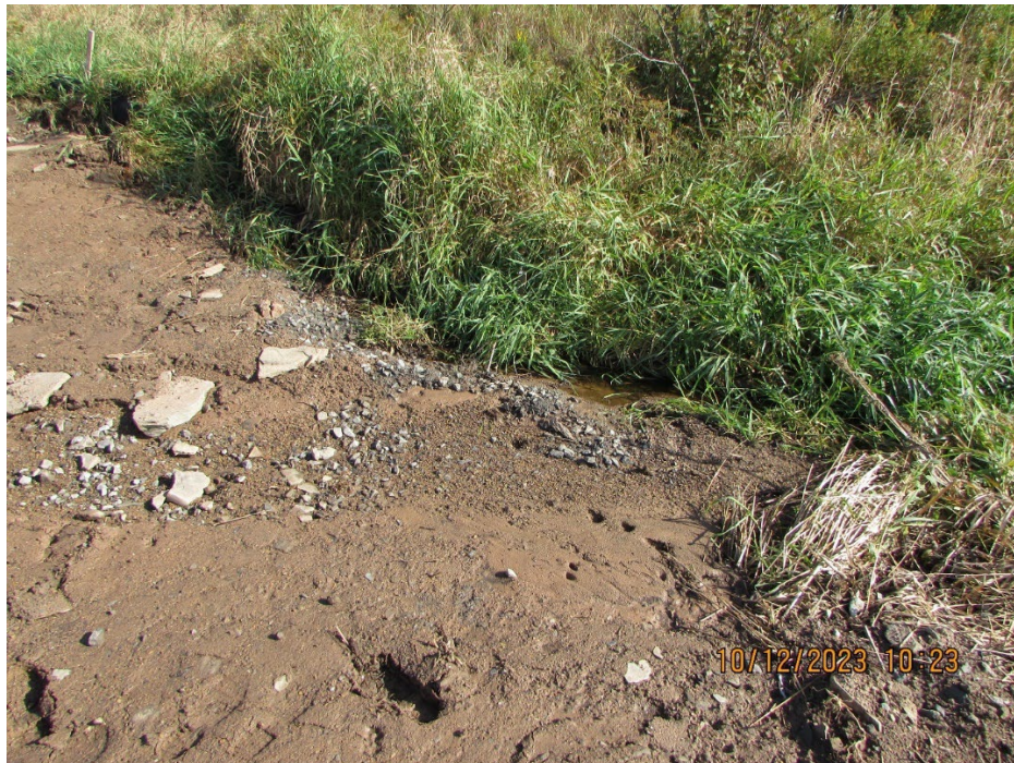
IMG 1618: view showing the drainage area for R-2. At the time of the inspection, the soil observed in this area was very wet and holding water.
