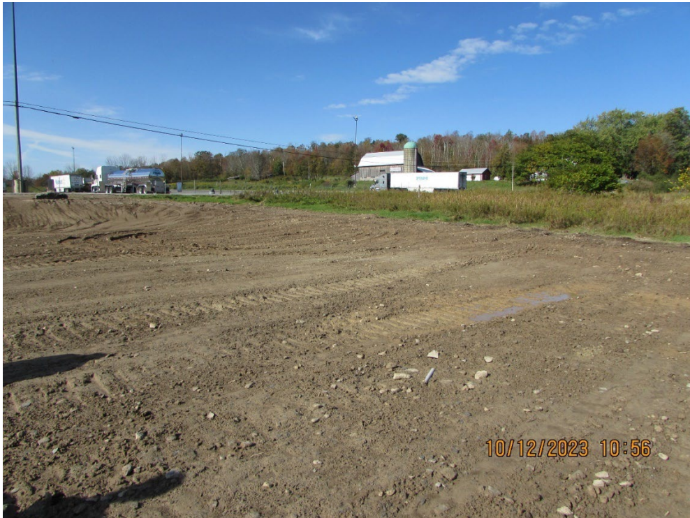
IMG 1629: View facing northwest. During the inspection, the Project Manager stated this area was not at the pre-disturbed grade because the pre-disturbed grade showed a significant drop in topography.
