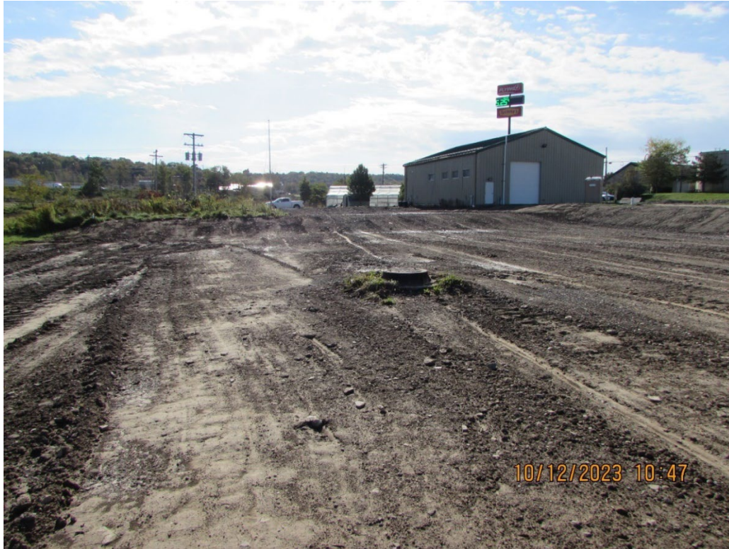
IMG 1626: View facing south within R-1. Closer view of the manhole.
