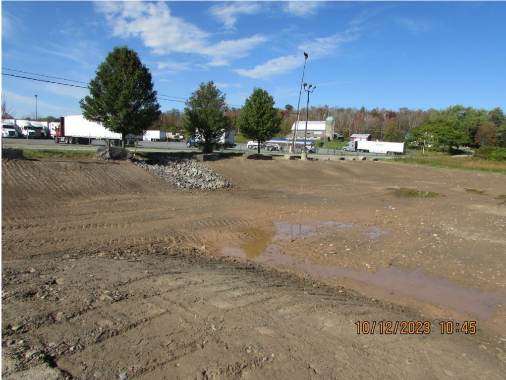
IMG 1624: View facing northwest showing R-1. Note the riprap that was put in place to carry stormwater from the adjacent road into the wetland.
