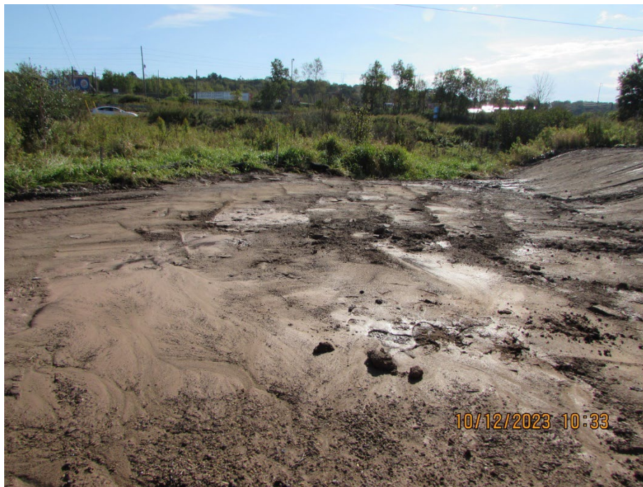
IMG 1621: View facing southeast of area R2. The soil in the northwest portion of R2, which is visible at the bottom of the picture above, was found to be compact at the time of the inspection.
