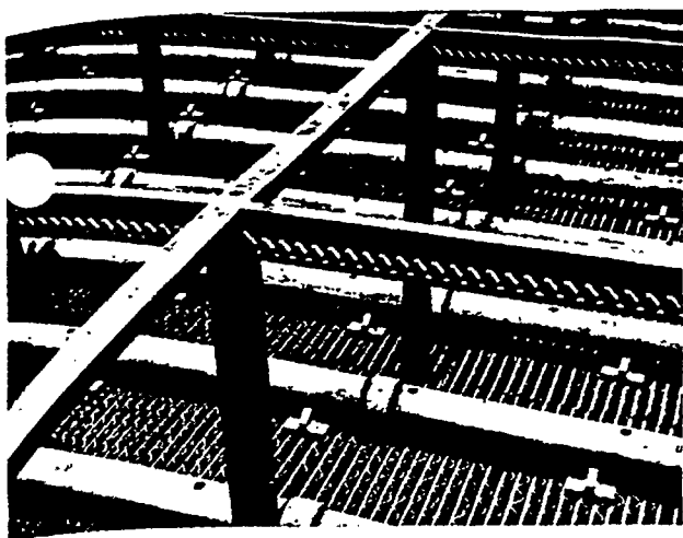
Fig. 4a—Top view of new cooling tower packing gives an excellent view of the many uniform flow paths possible for the air and water
