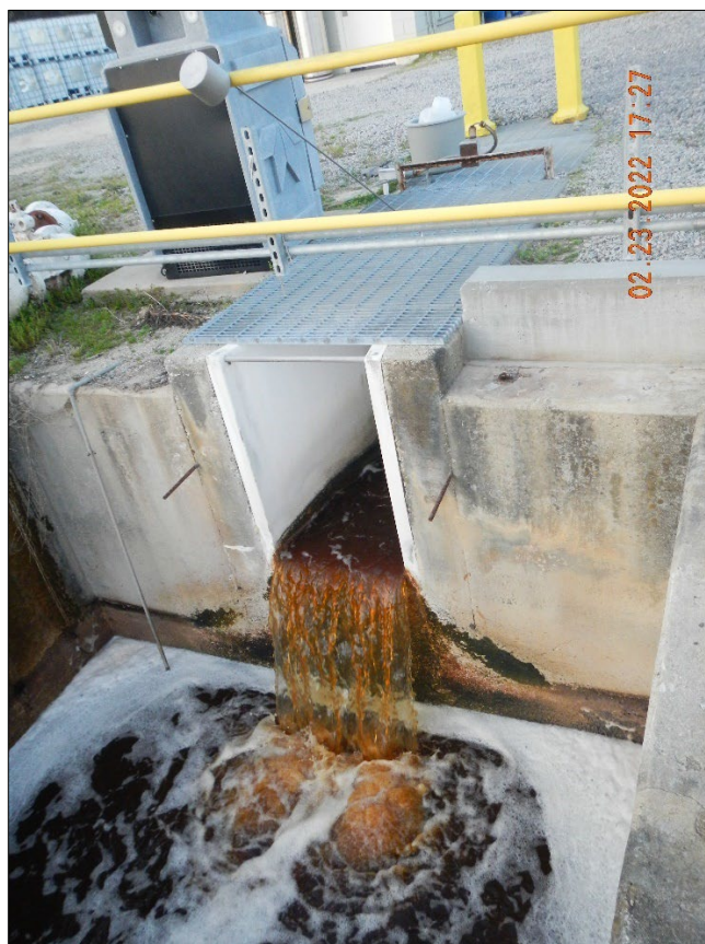
Photo-7. DSM Pretreatment - Effluent Flume Discharge
