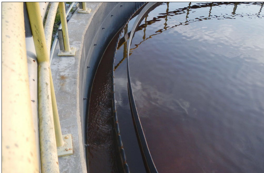
Photo-5. DSM Pretreatment - 8-FT Clarifier Overflow
