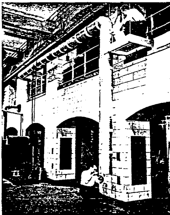
Pilot plant for stack dust sampling studies.
