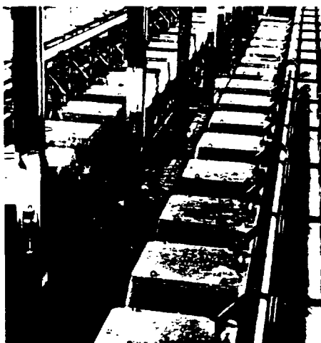
Salt brine is decomposed into chlorine and caustic cell liquor in electrolytic cells in a new production unit at the Baton Rouge plant.
