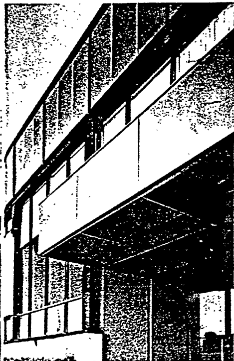
asbestos-cement sheets. Left: coloured sheets are used on balcony and soffit ceiling of an elegant marquee are covered
