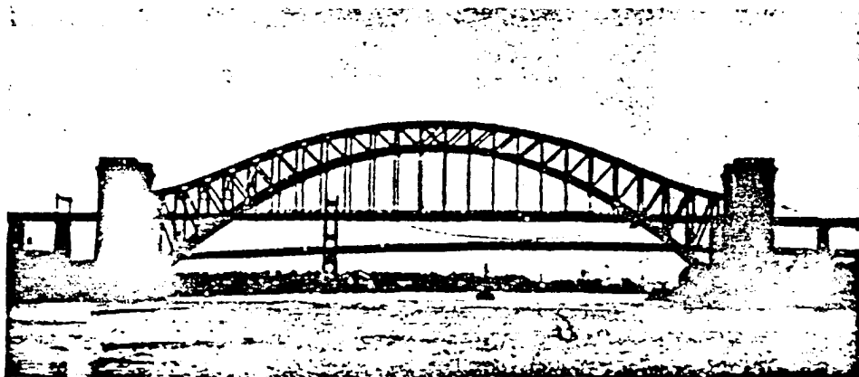
The steel work of the famous Hell Gate railroad bridge is protected against corrosion by a red lead base primer paint, another form of lead used extensively by the railroads
