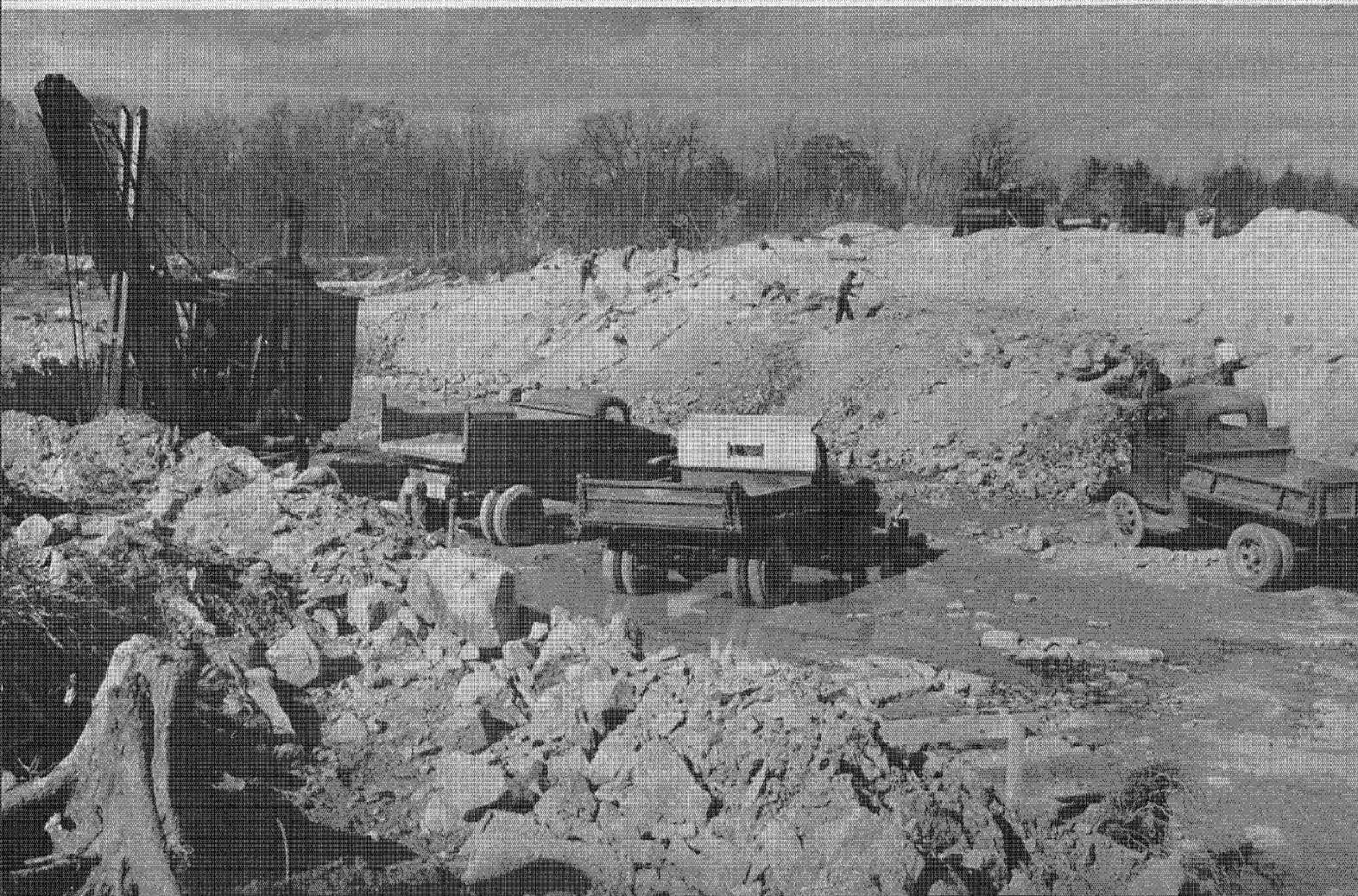
A typical construction view at an early stage of work. Rock ledges in northern sections kept blasters busy.
