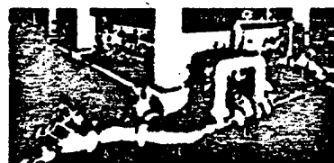
Shows Lead pipe line for handling a salt solution. Pipes are insulated to facilitate temperature control. Shows discharge pipe on the inside of a circular concrete mixing tank.
