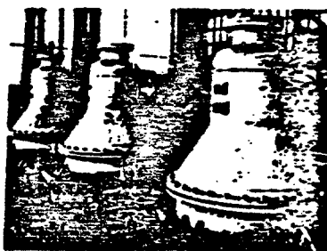
Above: Three homogeneous lead-lined steam apparatuses. Below: A homogeneous lead-lined tank. Homogeneous lead-lined units were installed in the tank.
