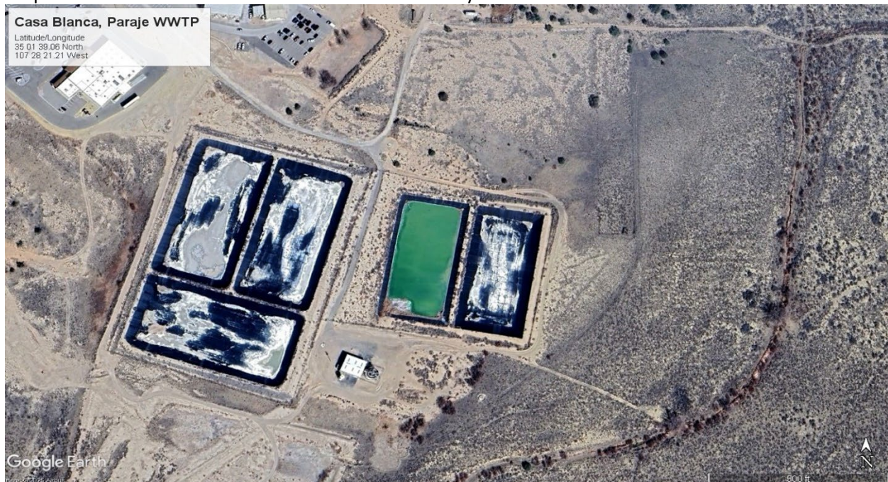
Aerial Image #1: Overall view of the Laguna Development Corporation- Casa Blanca Wastewater Treatment Plant location. Note: the evaporative lagoon cells. Aerial from Google Earth Maps.
