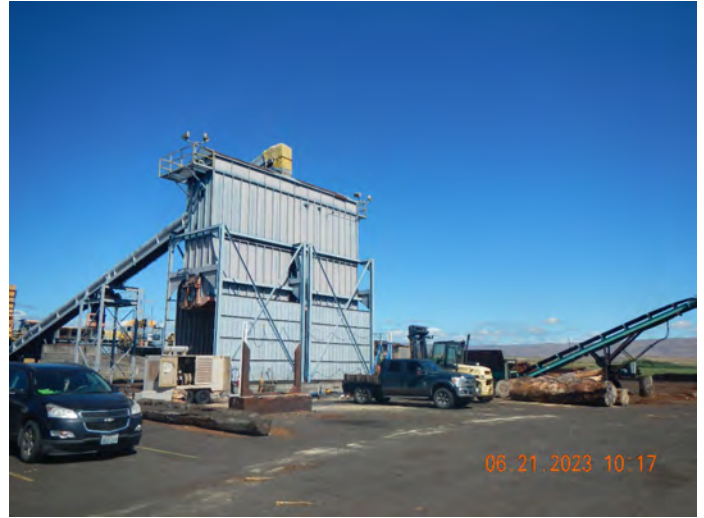
Photo #:06 (DSCN3295) Description: Facing northwest from the “large log mill,” photo of the hog fuel bin and conveyor located in the northeast portion of the mill.
