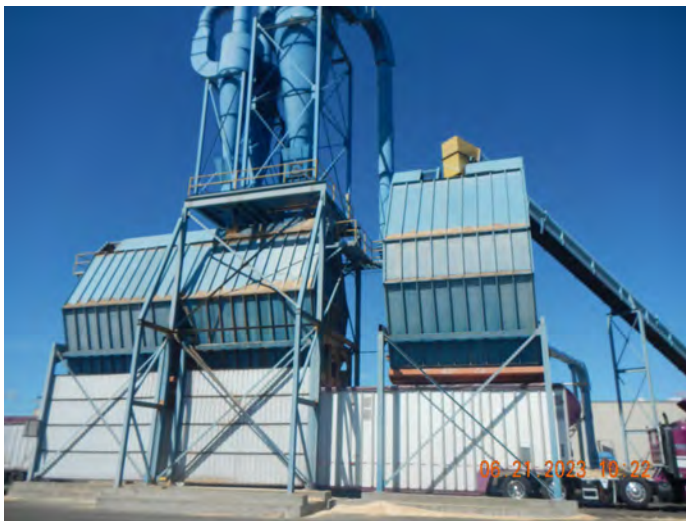
Photo #:07 (DSCN3296) Description: Facing west from the “large log mill” photo of the dry chip and shavings bins and conveyors.
