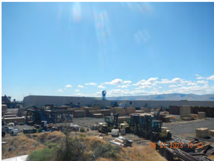
Photo #:17 Facing southeast from the “large log mill,” photo looking toward the mill and lumber storage area.
