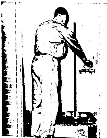
These built-in floor-level slop sinks installed in New York's Seagram Building are convenient and sanitary. At right, the roughed-in lead slop sink pan coated with asphaltum.
