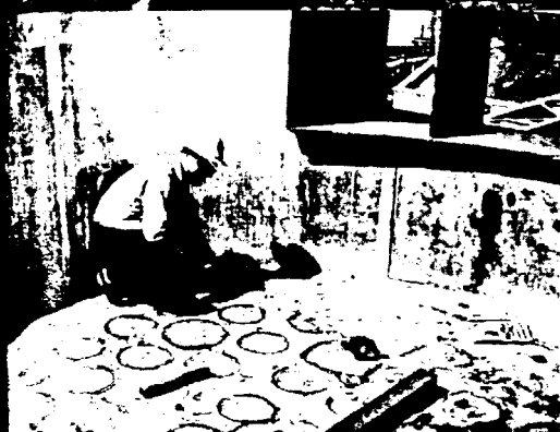
At left, 10-in. diameter holes for the precipitator tubes are being cut through the lead-lined floor of the upper chamber.
