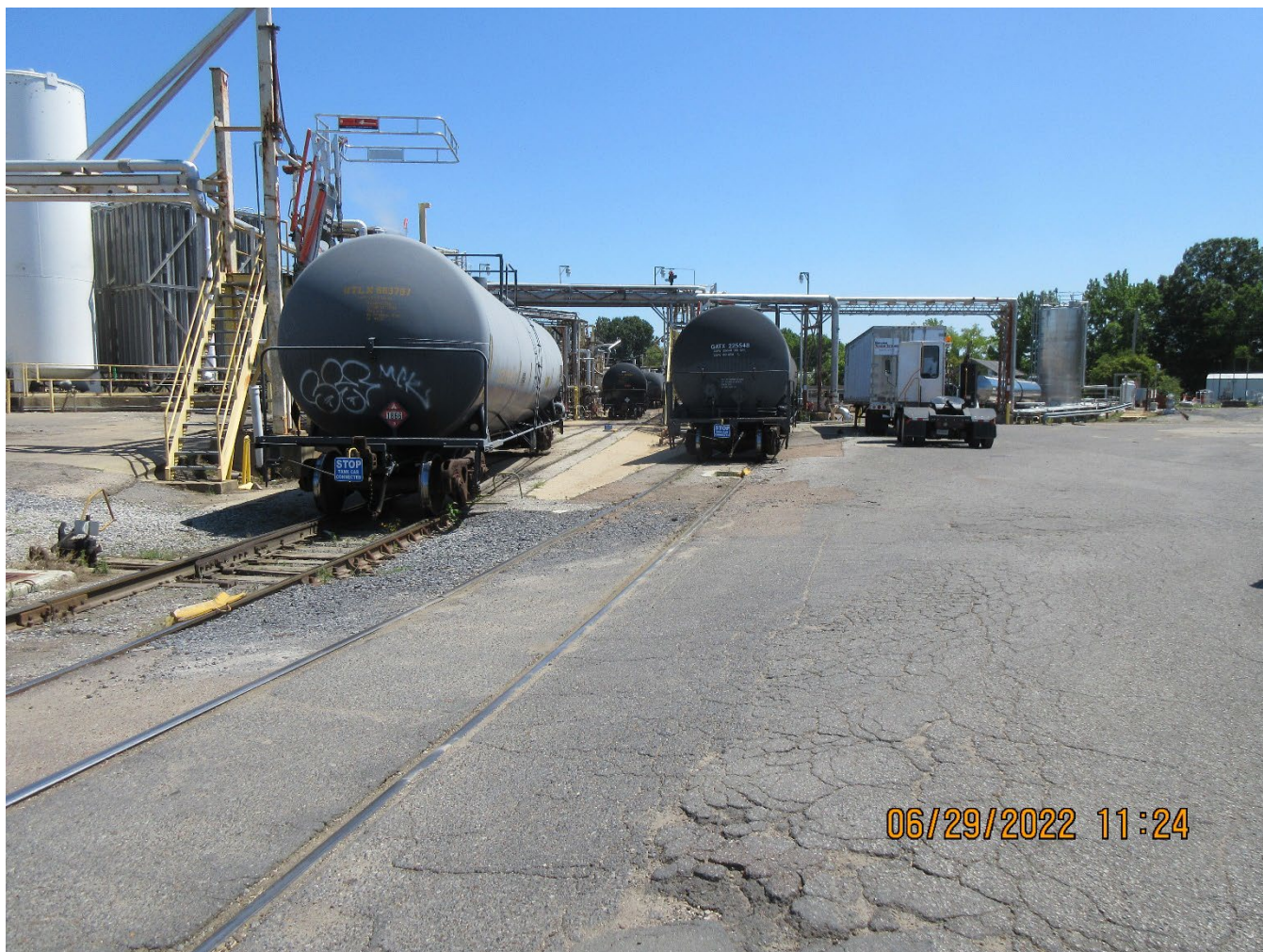
Photo 5 - Rail Spurs shown facility property in an off-loading area
