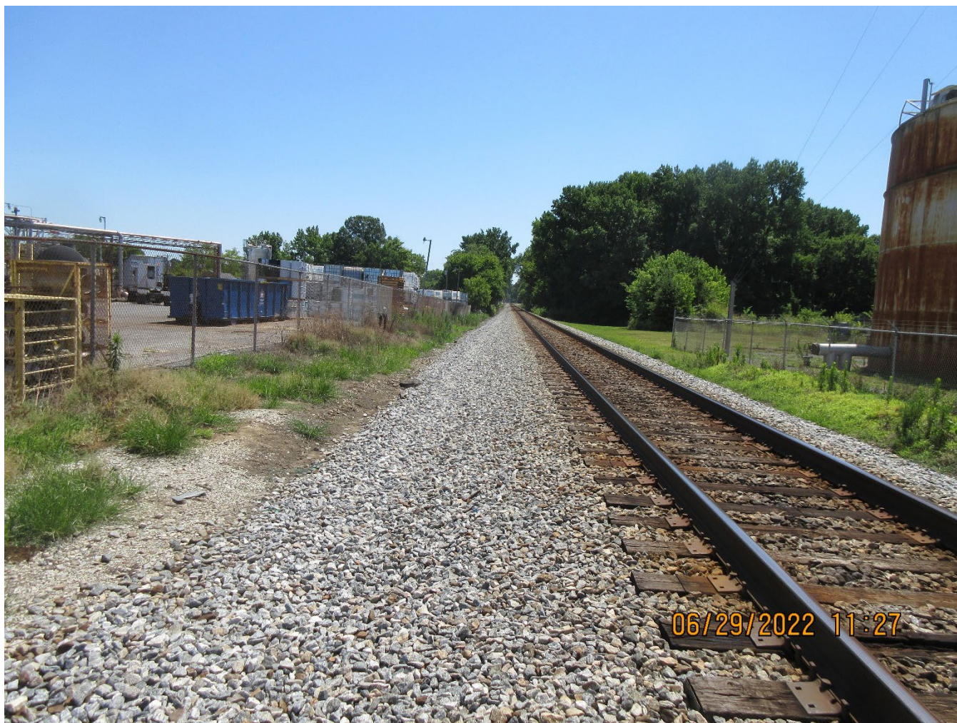
Photo 7 - Rail line running east/west through property
