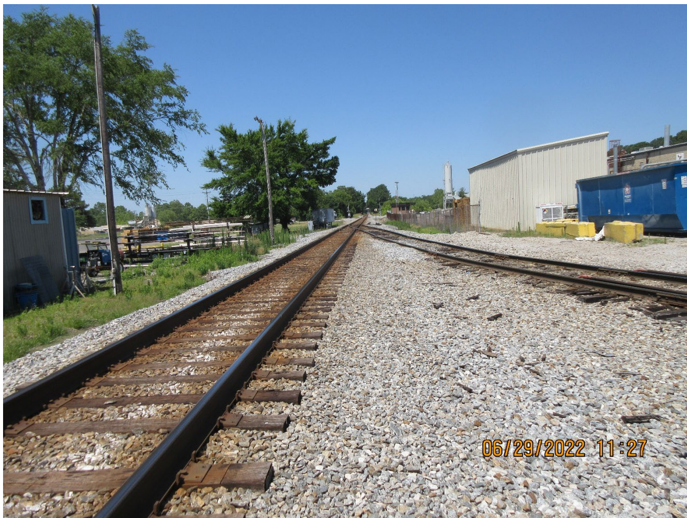
Photo 8 - Rail line running east/west through property with spur to AOC property
