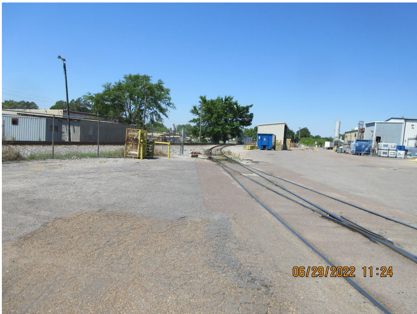
Photo 4 - Rail Spur shown (facing ESE) from rail line which dissects facility property
