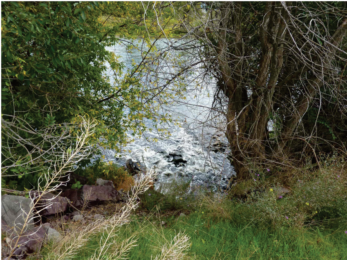
Figure 1 – POTW Discharge through Outfall 01 to the Clark Fork River
