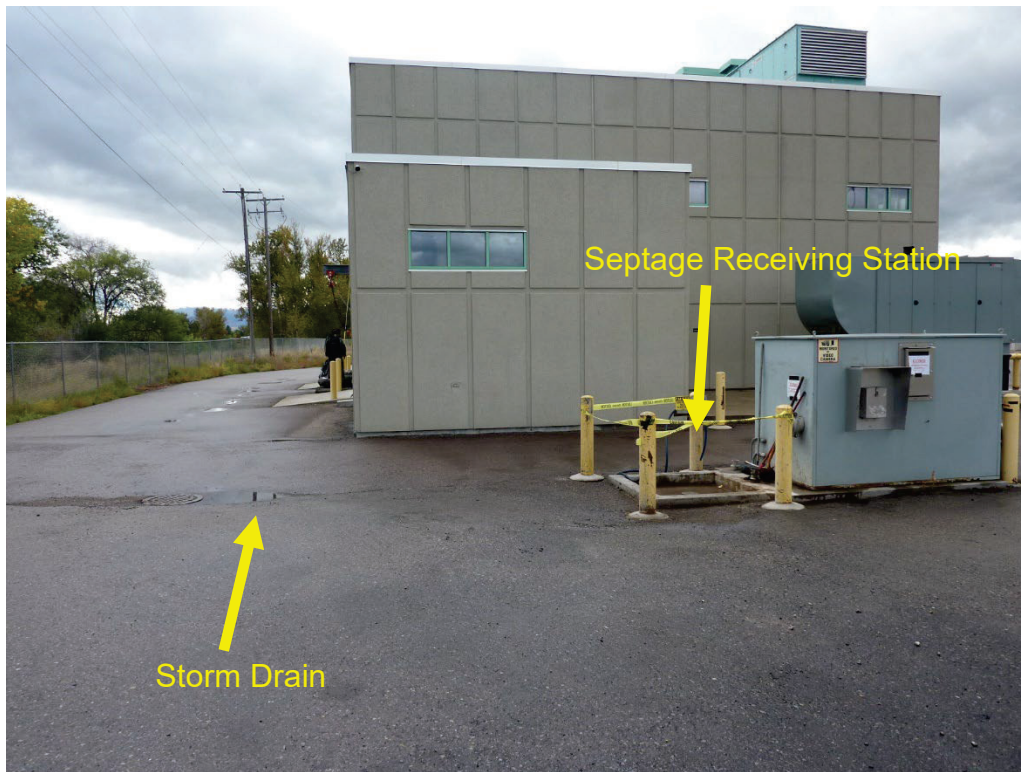
Figure 6 – Missoula Septage Receiving Station
