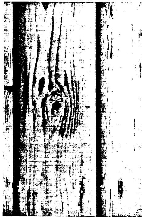
FIGURE 20.—Failure of paint over a knot that had been shellacked prior to painting.
