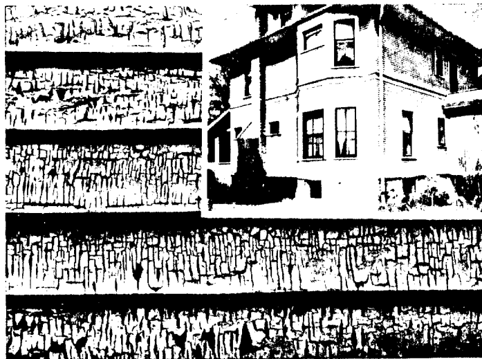
FIGURE 27.—Example of alligatoring.
