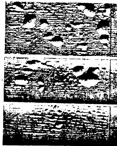
FIGURE 29.—Blistering of paint.
