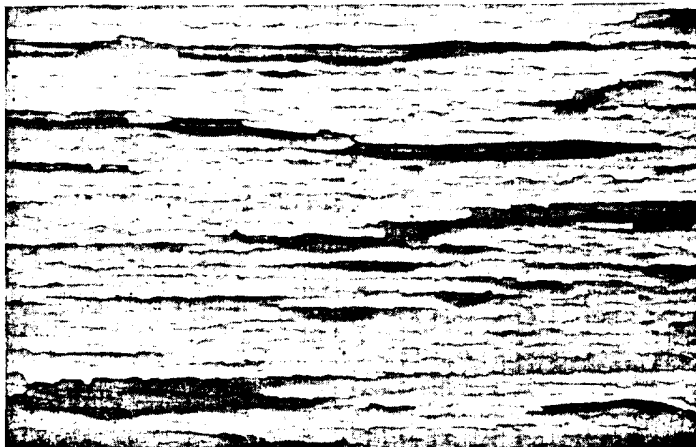
FIGURE 28.—Checking, cracking, curling, and flaking of paint on southern yellow pine.
