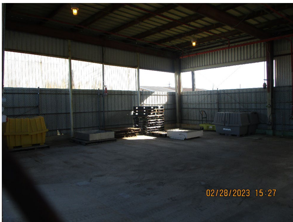
Photograph 19: Interior of mainly empty building.
