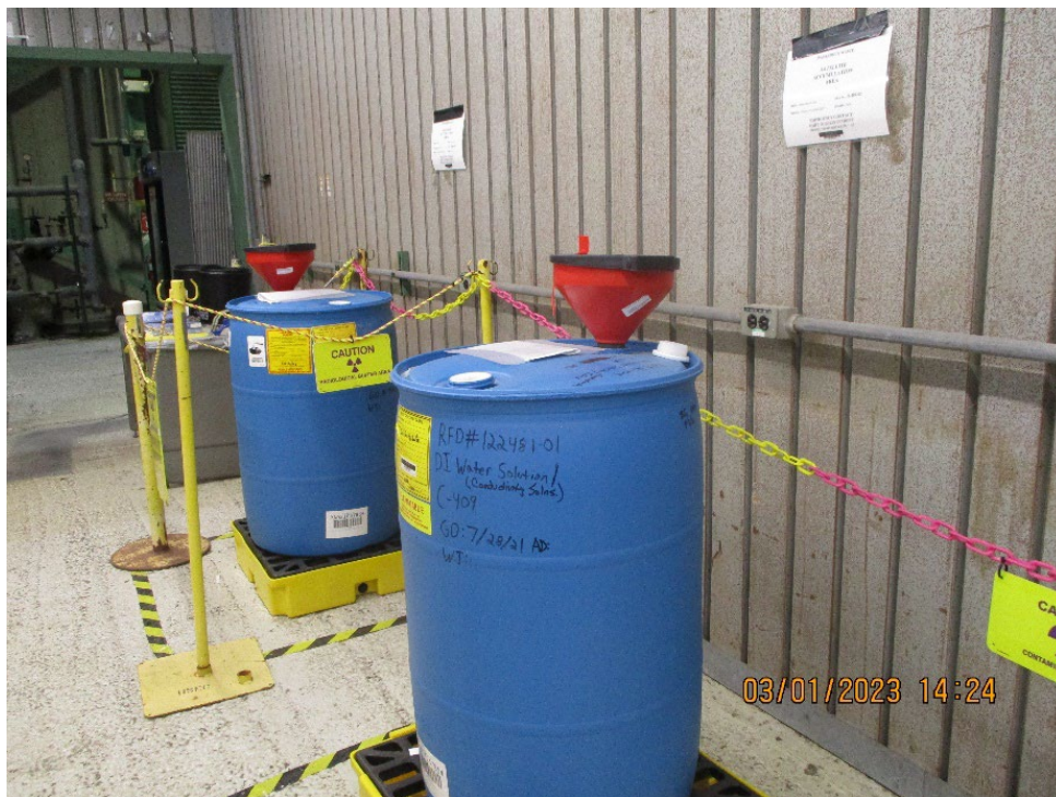
Photograph 62: Satellite Accumulation Areas in Building 409.
