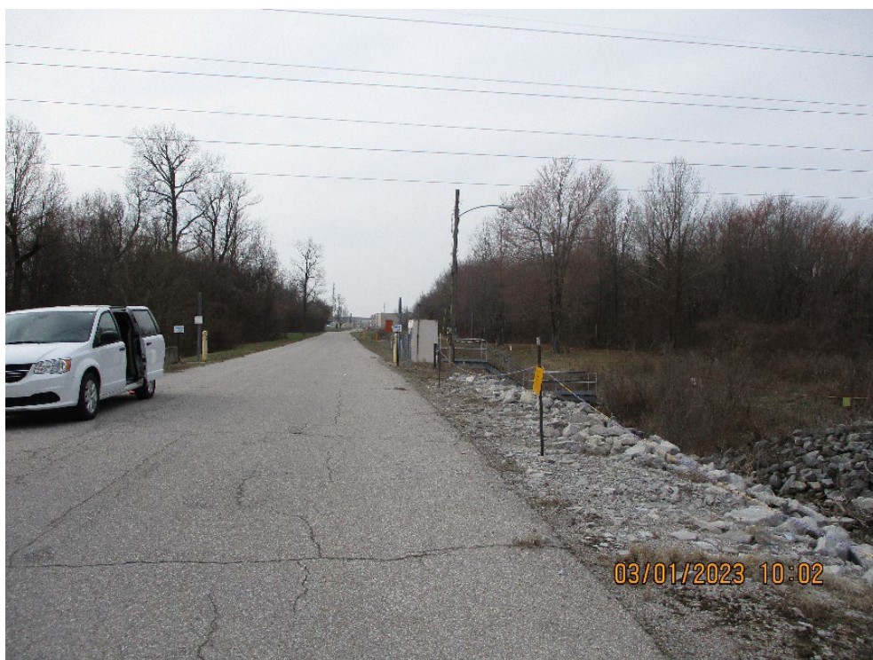
Photograph 74: Picture looking back towards the main facility from Ogden Road.
