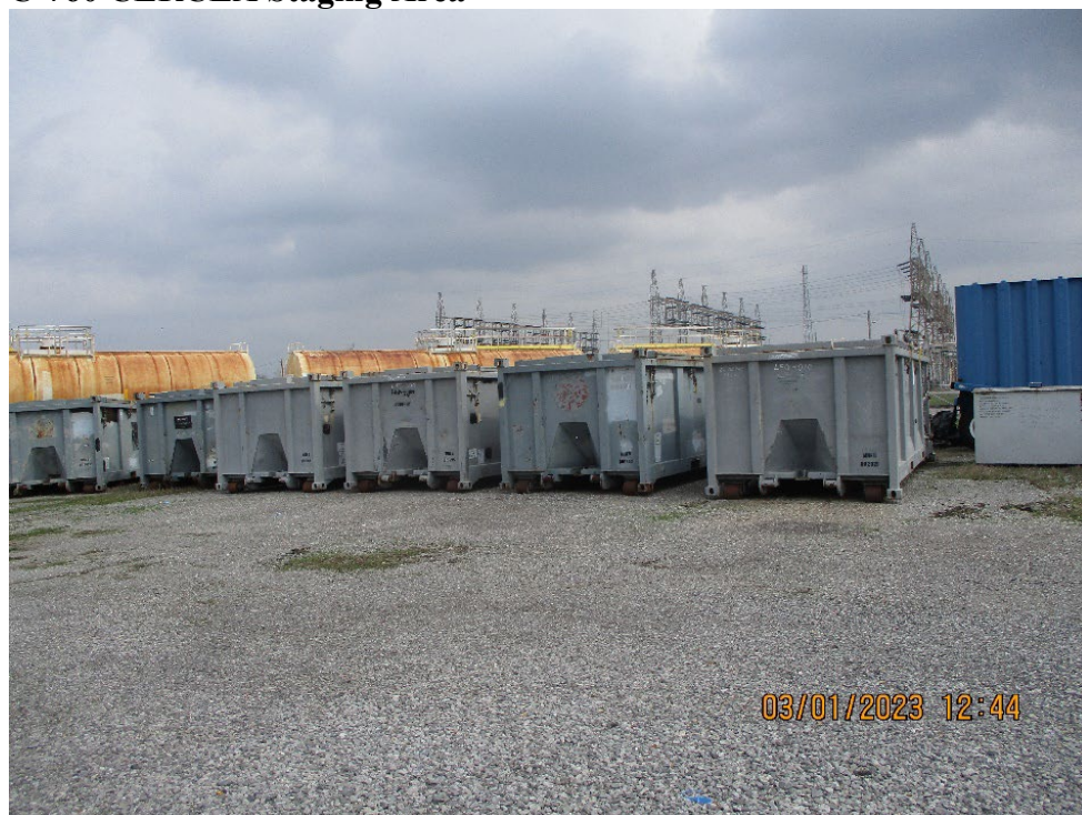
Photograph 39: Containers in the C-760 CERCLA Staging Area.
