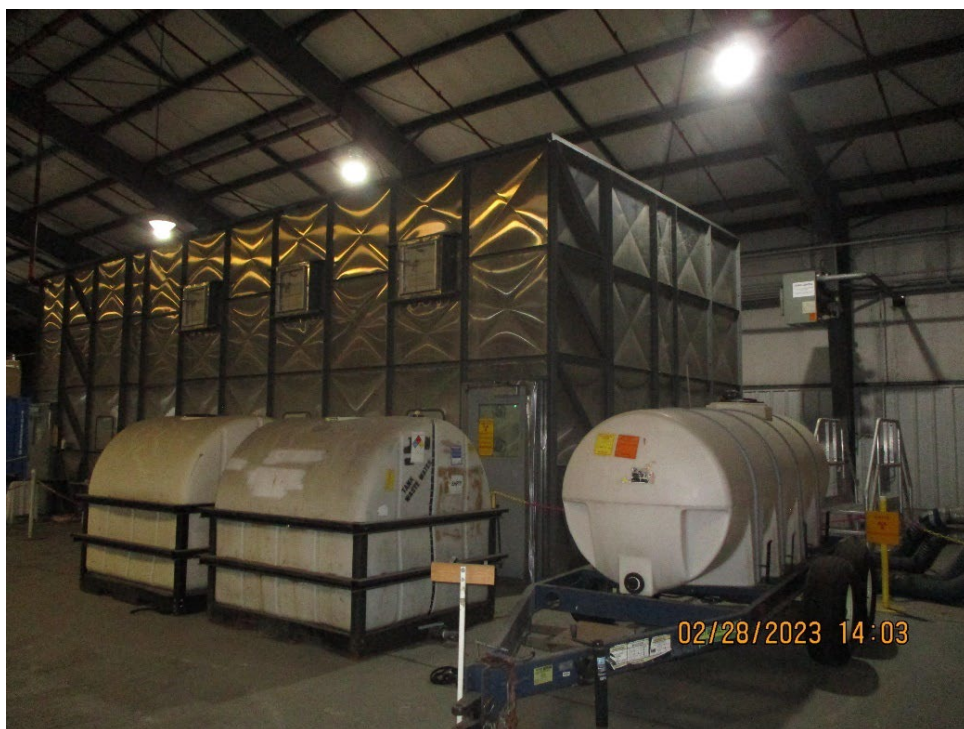
Photograph 7: Photograph of container work building (not in use).
