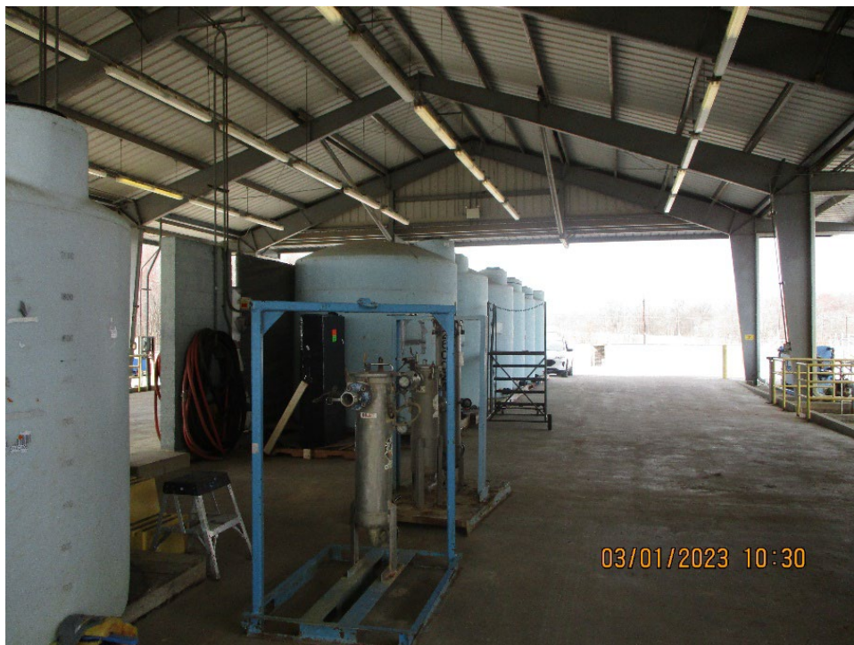
Photograph 33: Interior of C-752-C CERCLA Staging Area.
