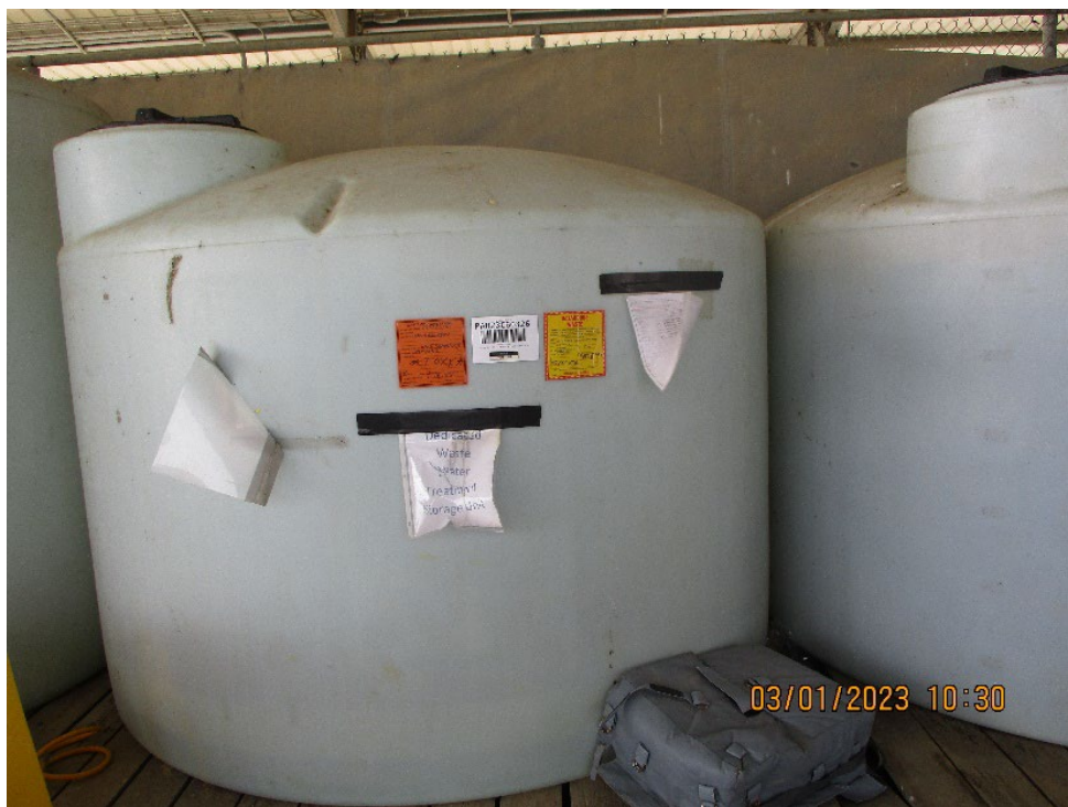
Photograph 35: Tank in interior of C-752-C with Hazardous Waste Wastewater.
