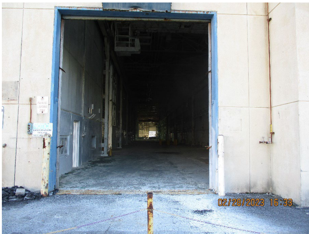
Photograph 31: Picture of empty interior of Building 400.
