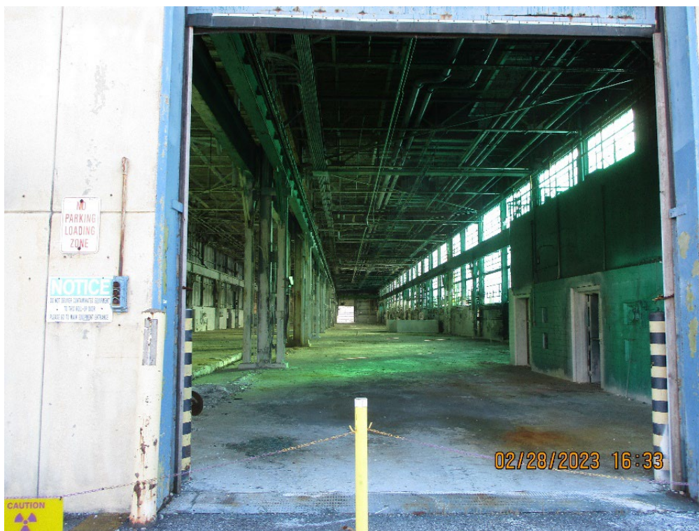
Photograph 32: Picture of empty interior of Building 400.
