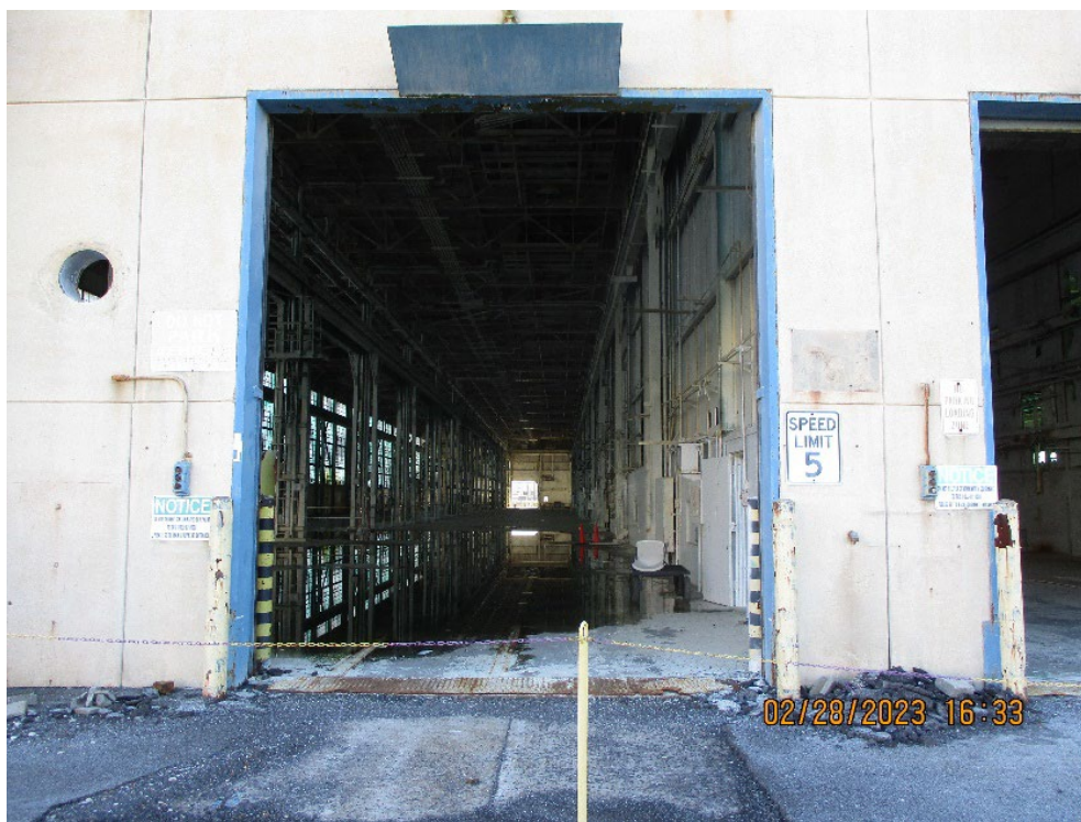
Photograph 30: Picture of empty interior of Building 400.
