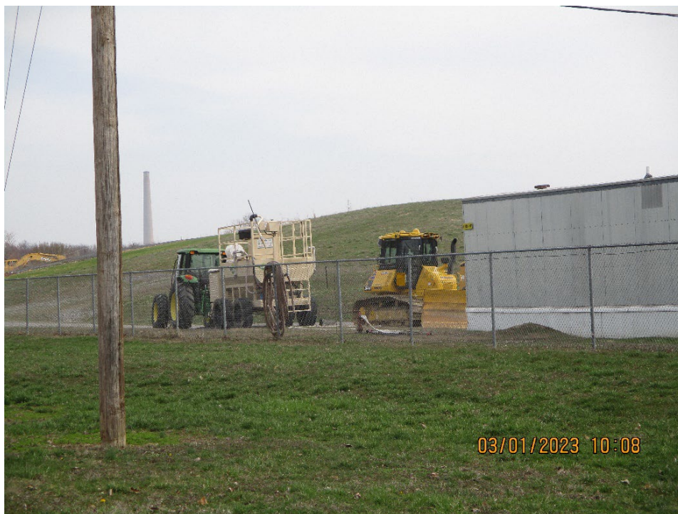
Photograph 78: Second picture of the landfill area.
