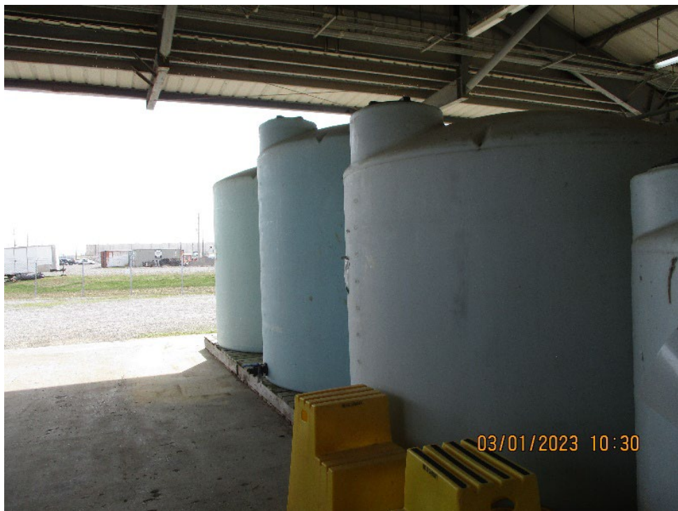
Photograph 34: Interior of C-752-C CERCLA Staging Area.
