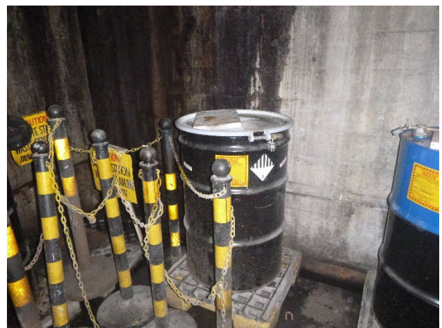
Photo 11: Coal Plant Powerhouse .
