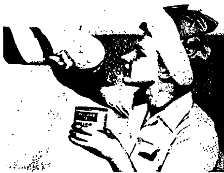
STRIPES painted around low overhanging pipes are a danger signal to help prevent head injuries when you're walking in the cellar.
