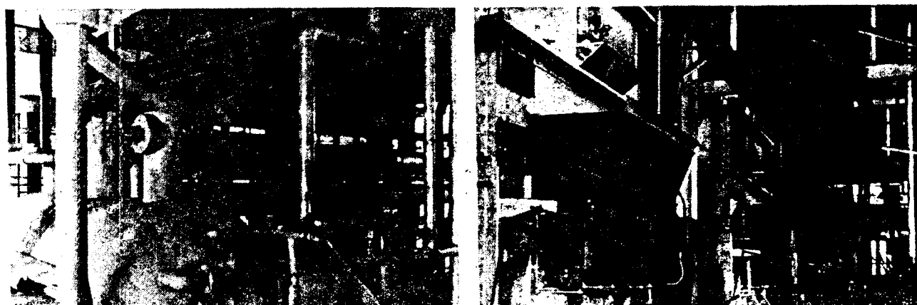
Fig. 6. Steam collection drum is insulated with 2 in. board insulation which is canvas covered, cement sealed, and painted. Steam is at 140 lb and 330 F. Mains are insulated with 1 in. formed pipe insulation and covered in the same manner as the drum insulation. Fig. 7—right. water at 180 F and is also insulated with 1 in. mineral wool blocks, covered with cement and paint
