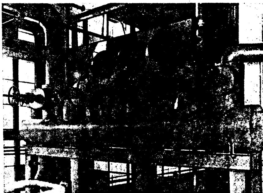
Fig. 6. Steam collection drum is insulated with 2 in. board insulation which is canvas covered, cement sealed, and painted. Steam is at 140 lb and 330 F. Mains are insulated with 1 in. formed pipe insulation and covered in the same manner as the drum insulation. Fig. 7—right. water at 180 F and is also insulated with 1 in. mineral wool blocks, covered with cement and paint
