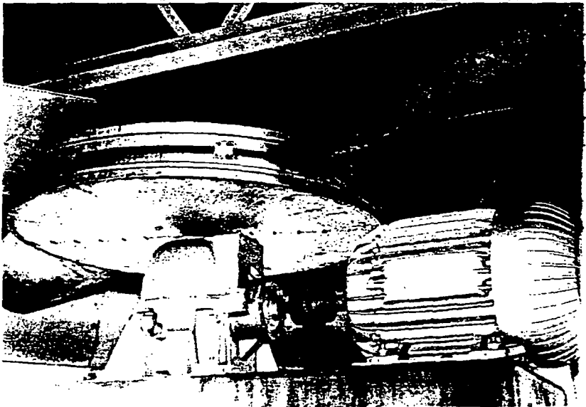
A 30-hp Sealedpower driving the "Fin-Fan" on the dehydration cooler. This drive is also representative of those used on the gas cooling "Fin-Fans."
