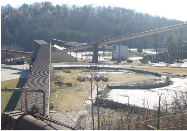
Photograph 12: Conveyor system from C&B Building to Kilns.
