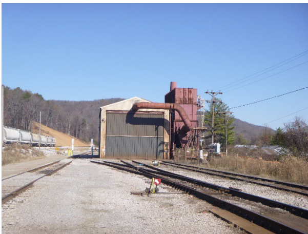
Photograph 2: Rail Yard - hopper car unloading area.
