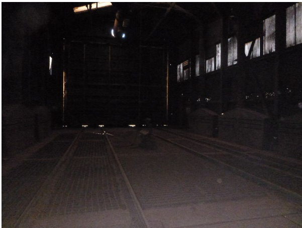
Photograph 3: Rail Yard - hopper car unloading area.
