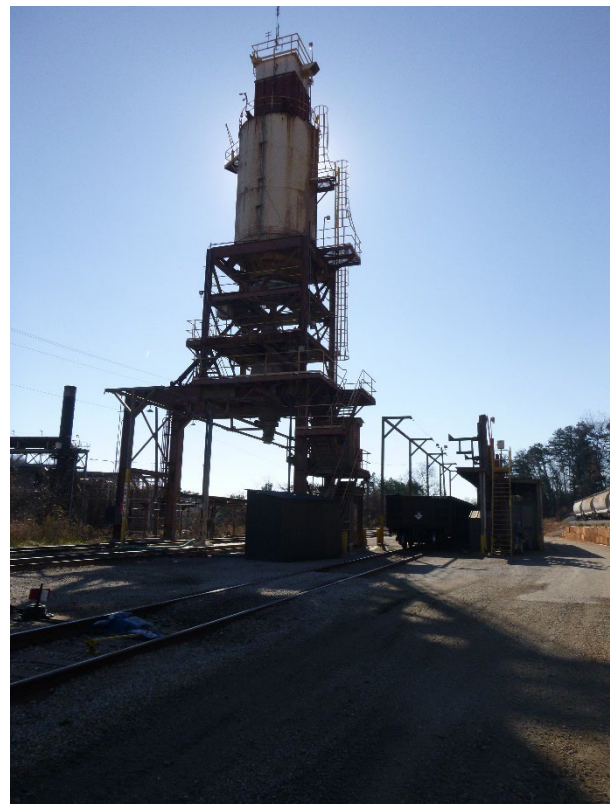
Photograph 5: Rail Yard – PD Railcar Unloading Area.
