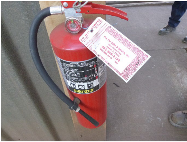
Photograph 6: Rail Yard fire extinguisher.
