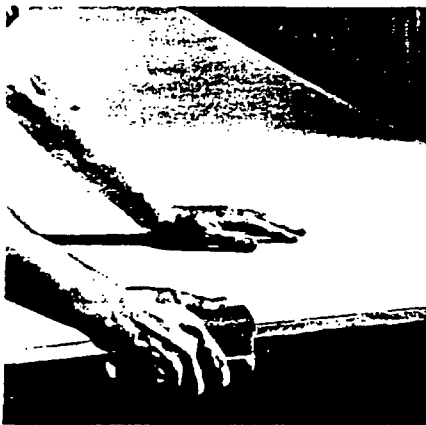
Smooth cut edges with a rasp, coarse sandpaper or metal lath wrapped around a block of wood, or trim with a cutting knife.
