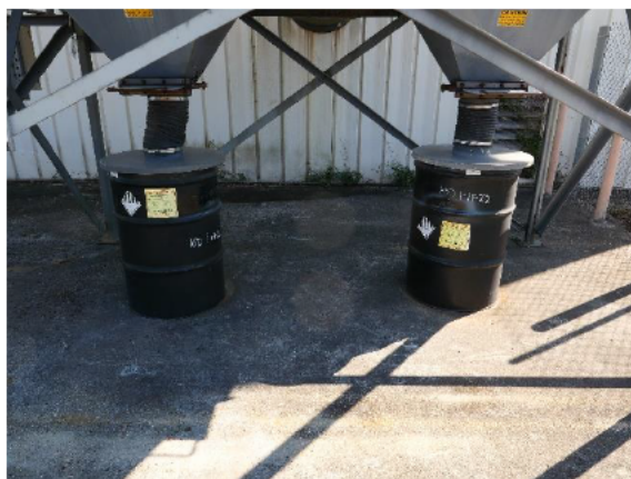
Photograph #2 - (b) (3) (A) spent plastic blast media container.
