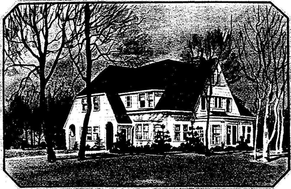
A stately country home in white, with red shingled roof.
