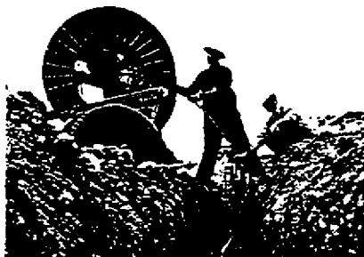
35-kv concentric neutral stranded aluminum conductor being installed to provide 3-phase service for commercial/industrial power loads.
