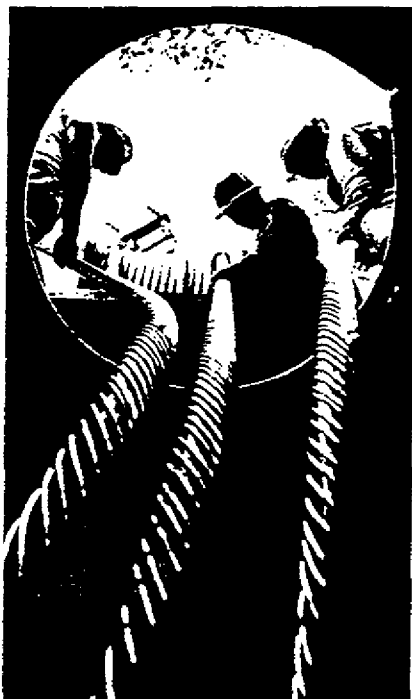
35-kv concentric neutral stranded aluminum conductor being installed to provide 3-phase service for commercial/industrial power loads.
