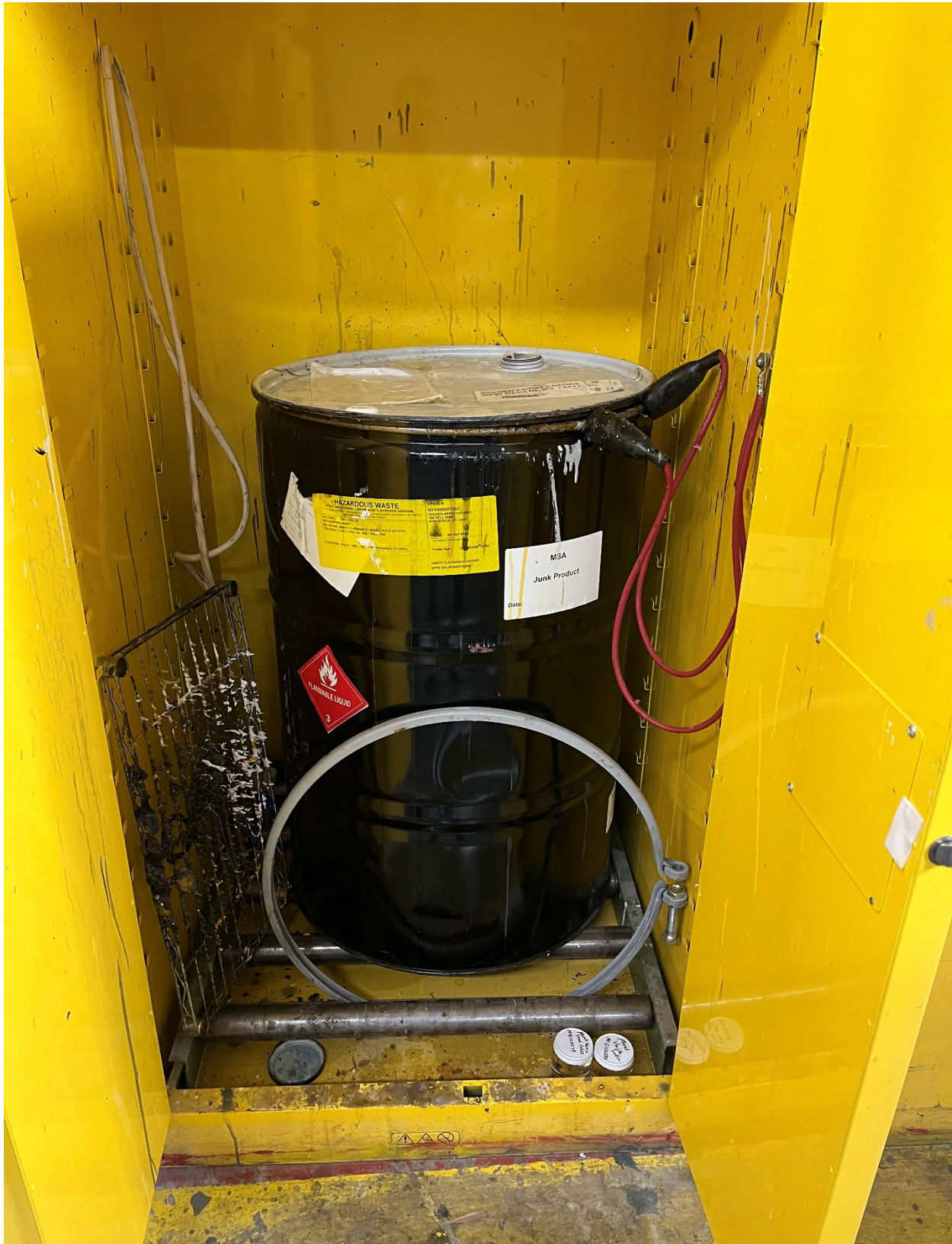
Photo #1: View of the satellite accumulation container for the liquid MSA waste.
