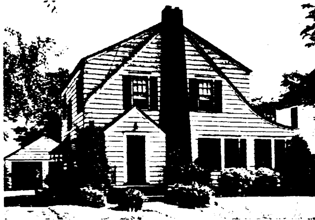
This house near Syracuse, New York, shows pure white lead paint still in excellent condition after seven years exposure to severe climatic conditions.
