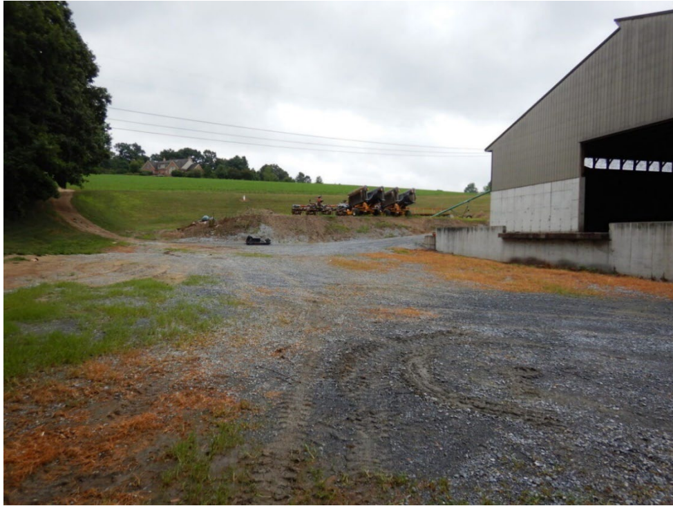
Photograph 11. View looking south at the area east of the manure storage building. Runoff from this area would flow into the swale located behind the photographer.
