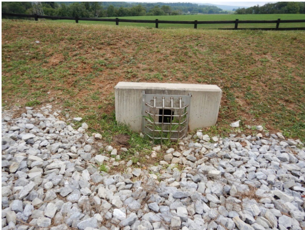
Photograph 28. Close-up view, looking northeast, of the outlet structure from the cattle housing stormwater basin located on the northeastern edge of the basin.
