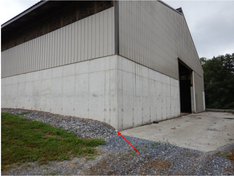
Photograph 7. Alternative view of the perforated drain with an unknown purpose (identified by the arrow) located at the southeast corner of the manure storage building.
