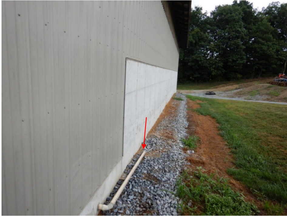
Photograph 5. Alternative view of the PVC pipe shown in Photograph 4 (downgradient view). The arrow indicates the outlet of the pipe where water would discharge into the gravel.
