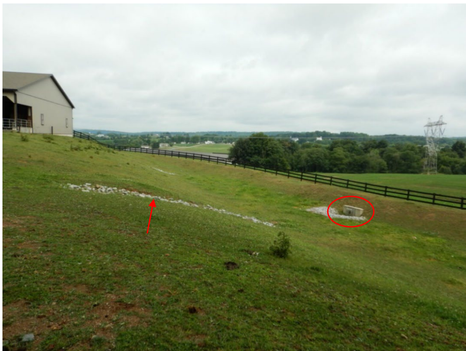
Photograph 24. View looking north over the cattle housing stormwater basin and pasture. The stormwater basin's outlet structure (circled) is located on the northeastern edge of the basin. A swale directing runoff into the basin is indicated by the arrow.
