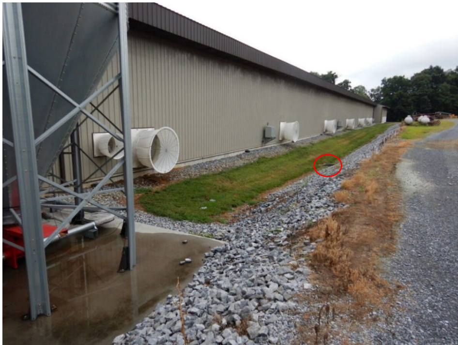
Photograph 2. View of the southern wall of the poultry barn (taken from the southwest corner of the building). The circle indicates the location of a storm drain that directs runoff to the poultry barn stormwater basin.
