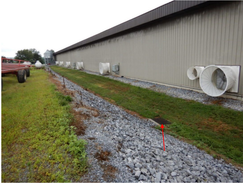
Photograph 3. Alternative view along the southern wall of the poultry barn (looking towards the feed bins shown in Photograph 2). The red arrow indicates the location of a second storm drain which directs runoff to the poultry barn stormwater basin.
