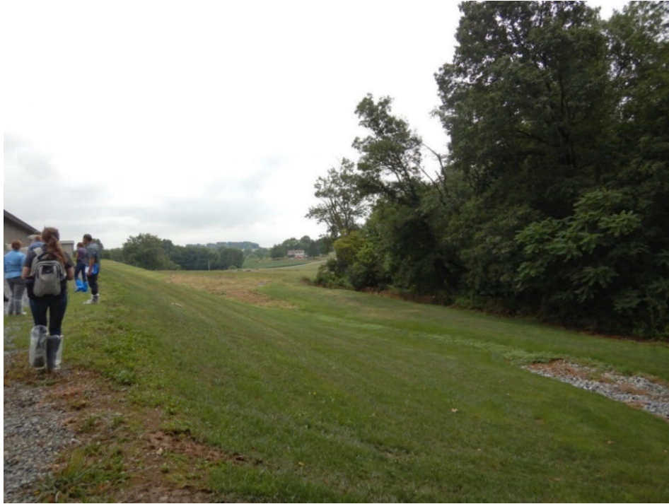
Photograph 13. View looking northwest at the stormwater basin located north of the poultry barn and manure storage building. Note the swale (shown in Photograph 12) at the right side of the photograph. This photograph was taken from approximately the same location as Photograph 12.
