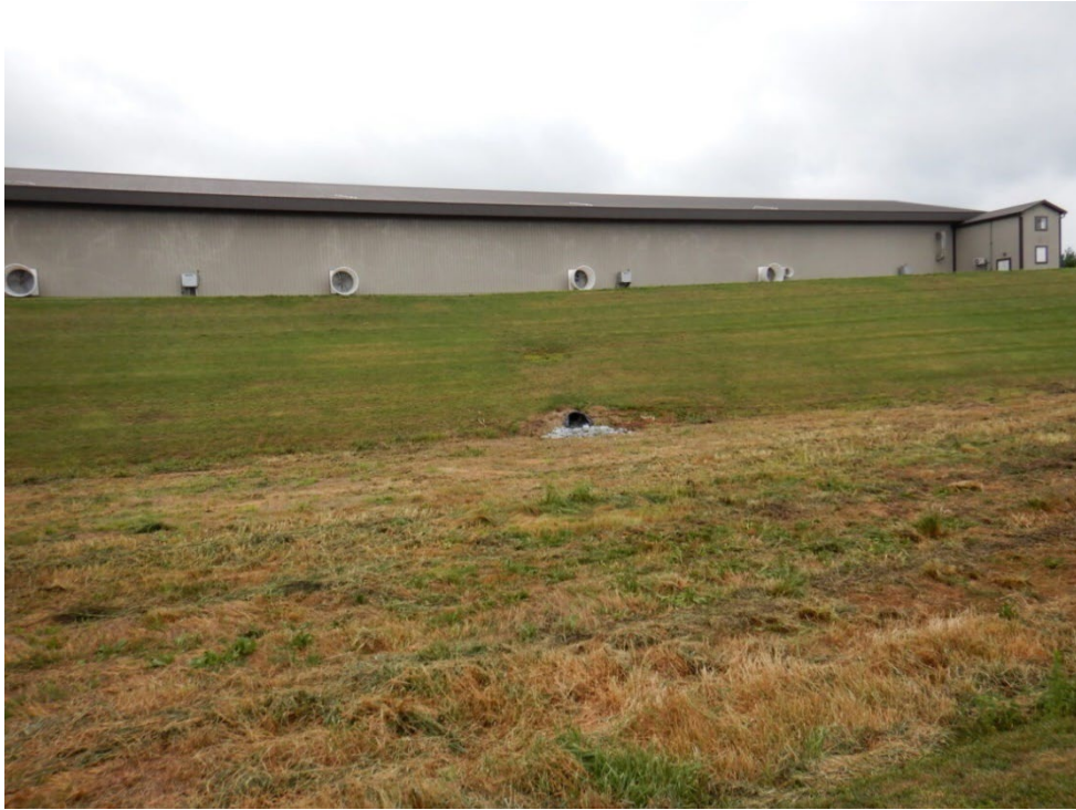
Photograph 19. View of the inlet to the poultry barn stormwater basin from the storm drain circled in Photograph 2.
