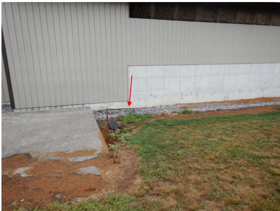
Photograph 4. The arrow indicates a PVC pipe located along the southern wall of the poultry barn. The PVC pipe conveys washdown water out of the building from the sump located beneath the concrete pad at the left side of the photo.
