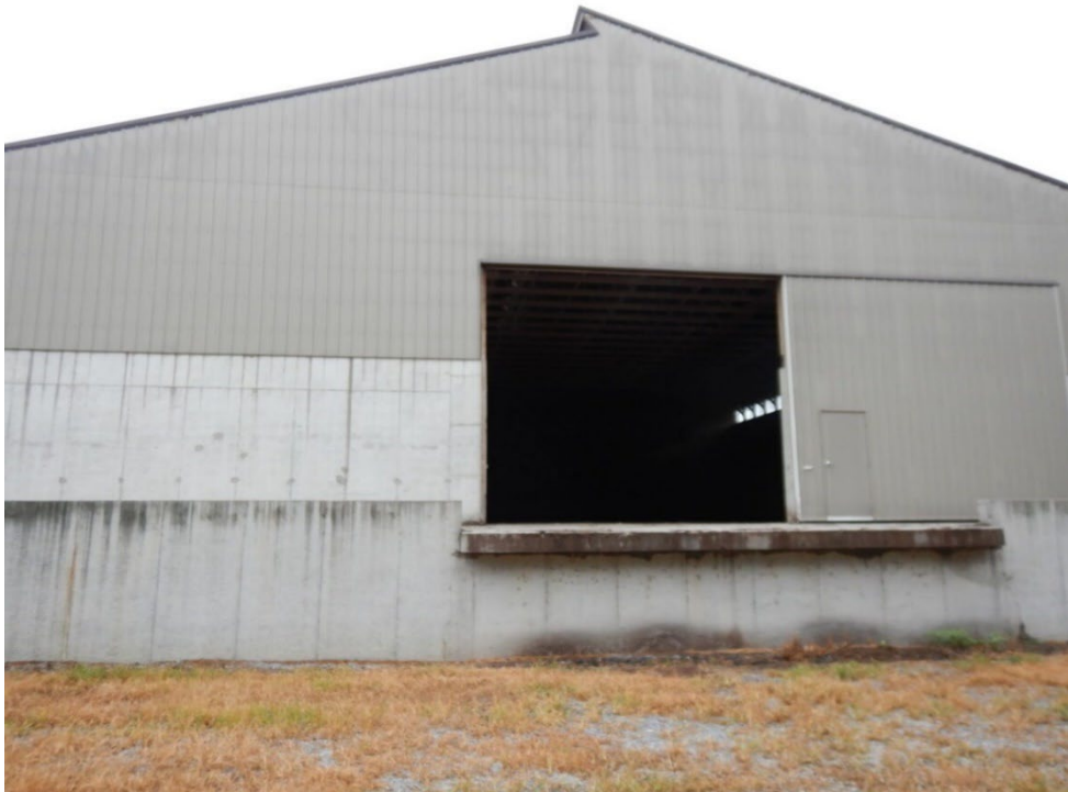
Photograph 8. View of the eastern side of the manure storage building and concrete pad.
