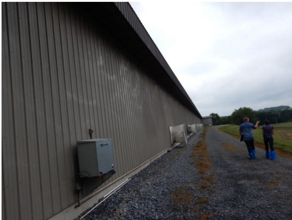
Photograph 14. View along the north side of the poultry barn (taken from the northeast corner of the building).
