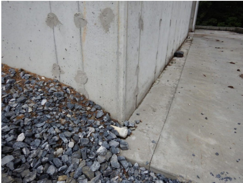
Photograph 6. View of a perforated PVC pipe with an unknown purpose located at the southeast corner of the manure storage building.
