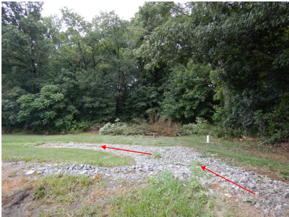
Photograph 12. Runoff from the areas shown in Photographs 10 and 11 would flow into the swale shown here (the arrows indicate the direction of flow). This photo faces north from approximately the same location as Photograph 11.
