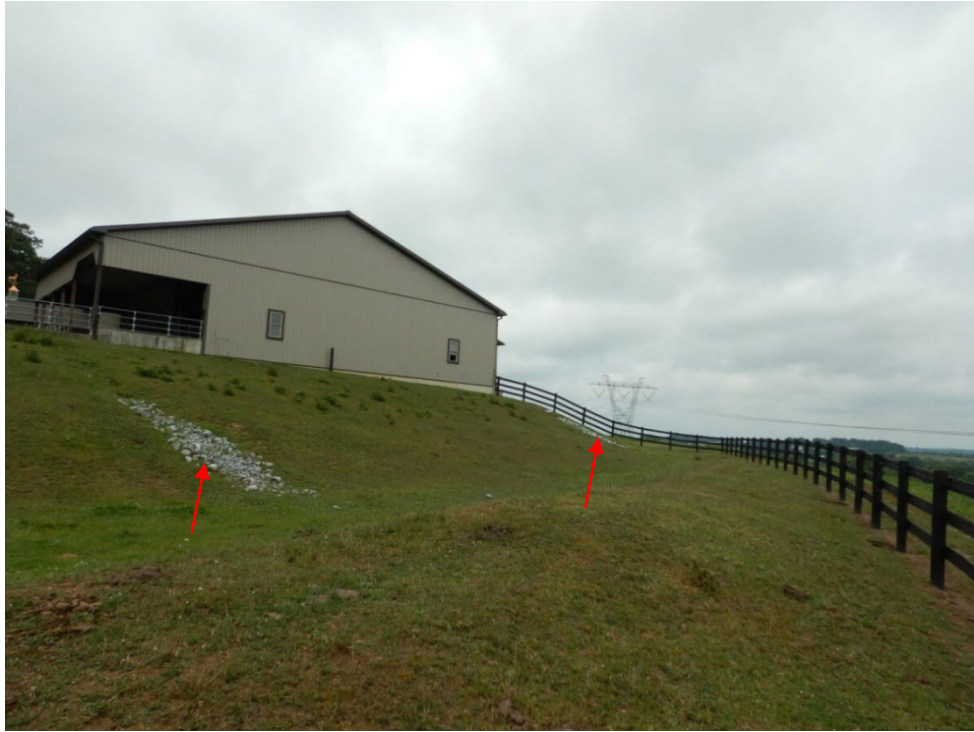
Photograph 27. View of the northern end of the cattle housing stormwater basin and swales (indicated by the arrows) feeding the basin.
