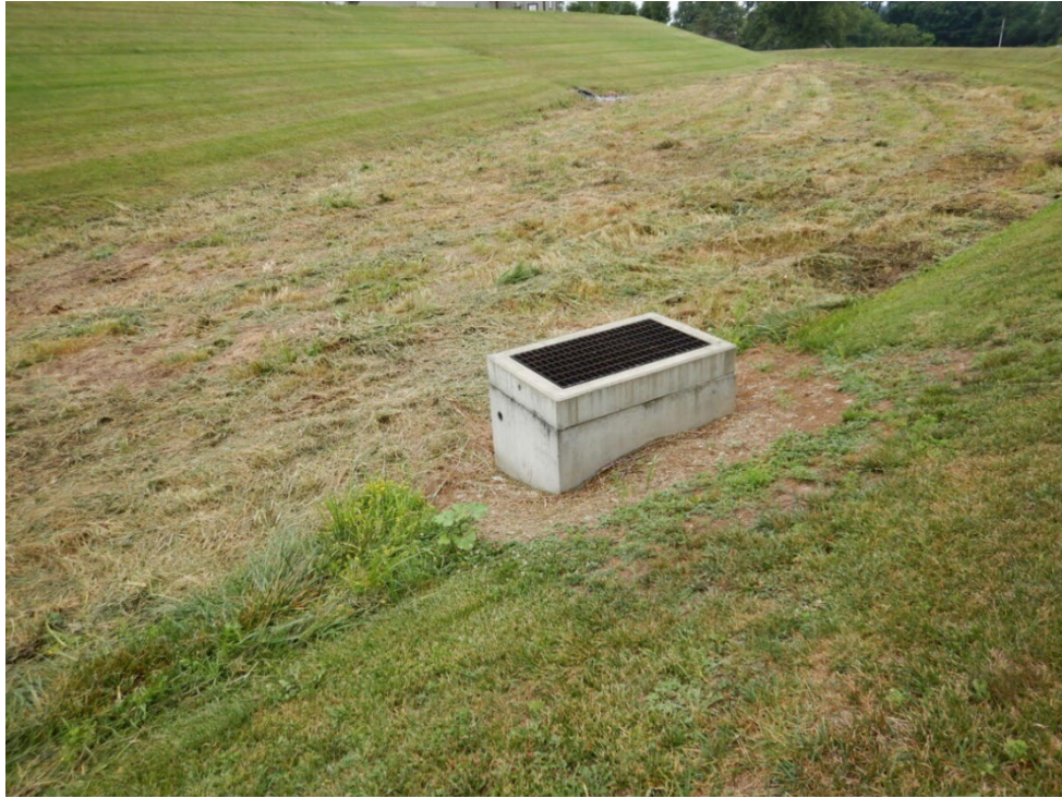
Photograph 17. Close-up view of the overflow structure located in the poultry barn stormwater basin, view looking west.
