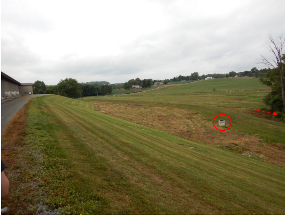
Photograph 15. View looking northwest over the poultry barn stormwater basin located north of the barn and manure storage building. The overflow drain is circled and the location of the unnamed tributary to Brubaker Run is identified by the arrow.
