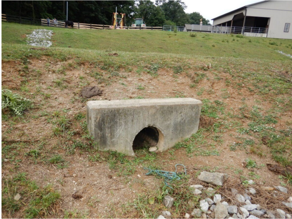
Photograph 25. Viewing looking southwest at the outlet from the cattle housing area stormwater basin with the cattle pen visible at the top right corner of the photograph.
