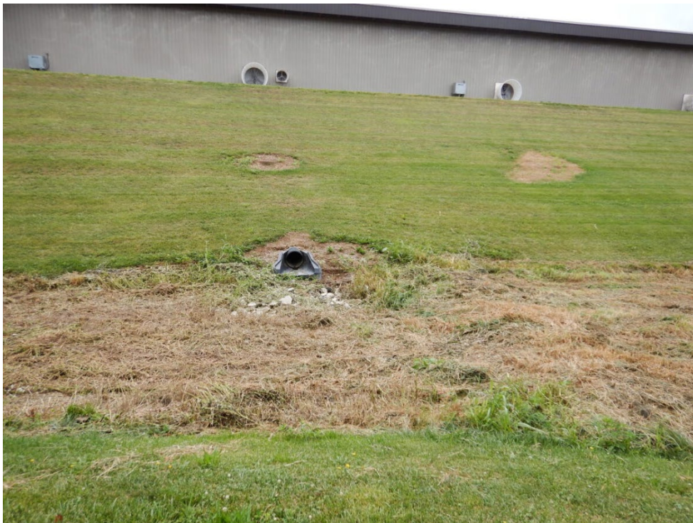
Photograph 16. View of the inlet to the poultry barn stormwater basin from the storm drain shown in Photograph 3.
