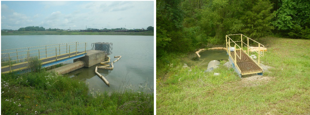
Figure 1: Left – Pond & discharge weir. Right – Effluent from Pond prior to flow measurement.
