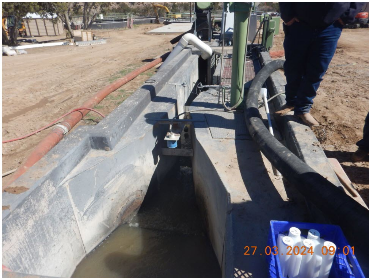
View of existing headworks looking approximately North. Note: this structure is identified in Appendix 2 Current White Rock Site Plan to be demolished or abandoned. (DSCN2688). Photographed by D. Esparza
